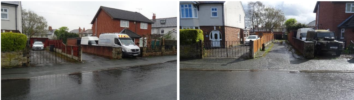
Figure 4.7. Access from road in 2022 (left) and 2024 (right)
