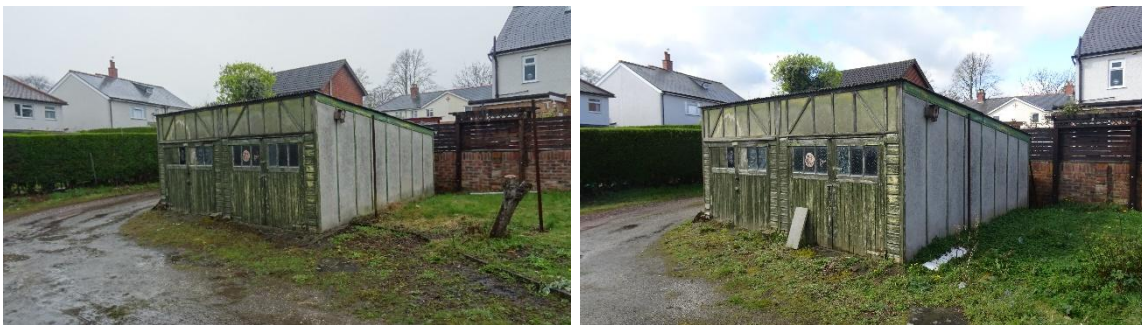
Figure 4.4. Detached garage building in 2022 (left) and 2024 (right)
