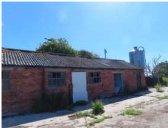
Front elevation wall
