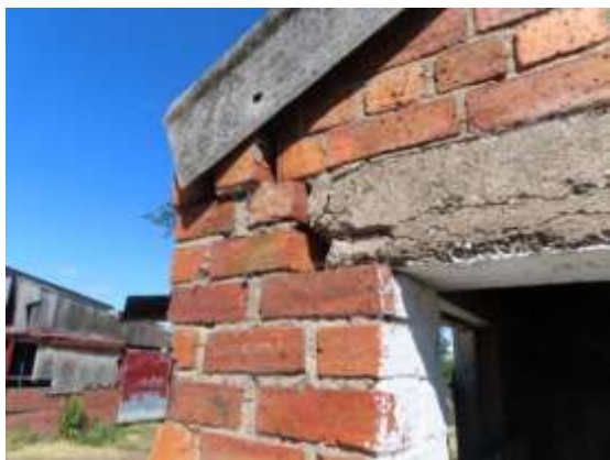
Dislodging brickwork
