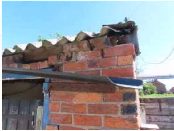
Disconnected gutter
