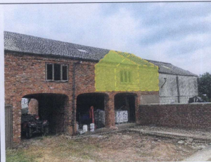
Plate 1: The western aspect of the Site. Note the brick building B1 and the cladding/blockwork building B2. Location of upper floor room shown highlighted yellow.
