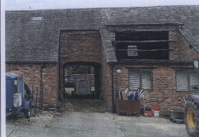
Plate 8: Eastern aspect. Large opening into adjoining building shown that allows access into B1.
