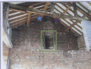
Plate 5: The 'open doorway' (outlined green) providing free flight access to B1 from the remaining building complex outside the redline boundary, and entrance to Roost R7 and R4. Blue star indicates location of Roost R6 and purple star Roost R10.
