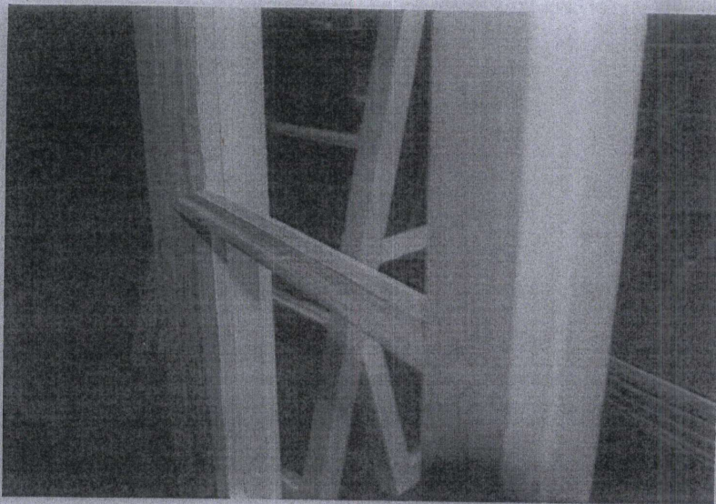
Figure 4 Moulding Profile for Replacement Windows.
