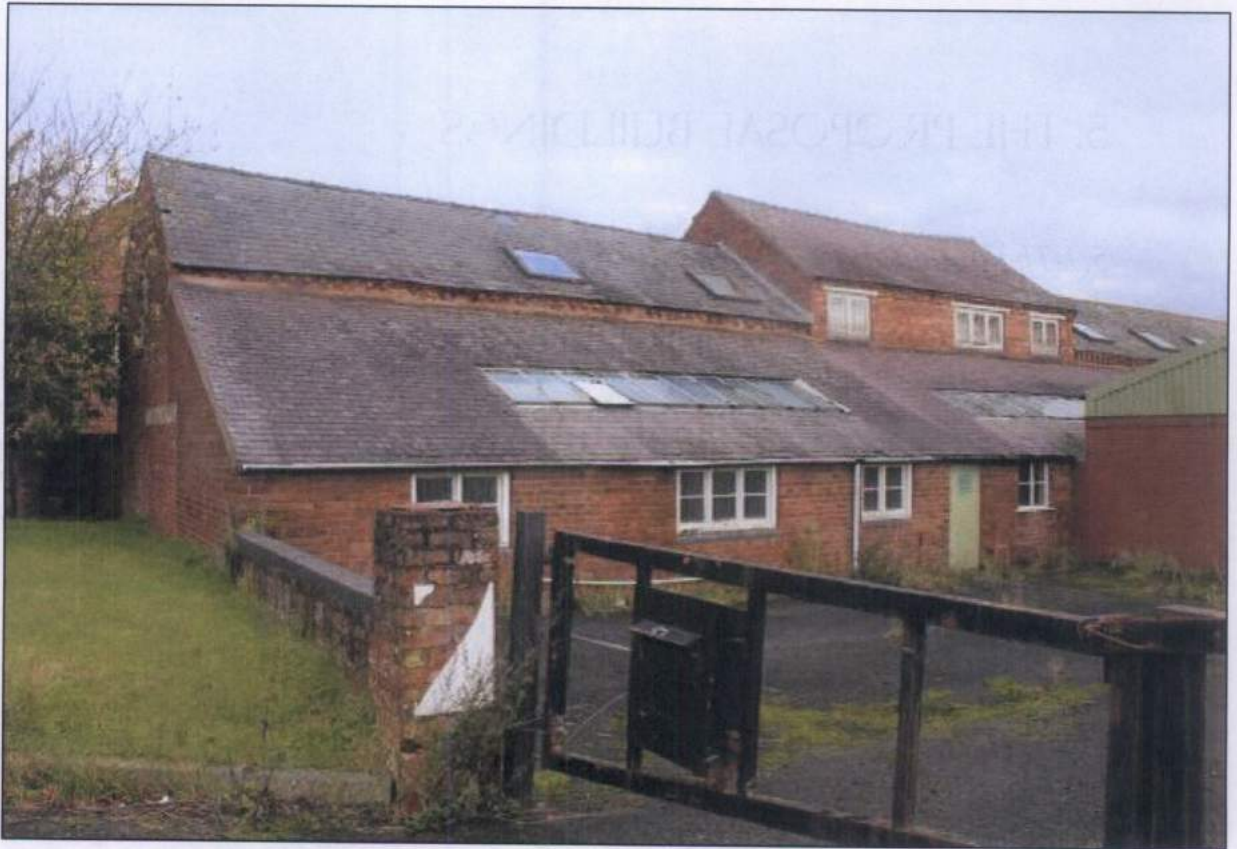
5. The single-storey outrigger at the south end of the west-east range, which is the element attached to the application building, is probably mid-20 th century
