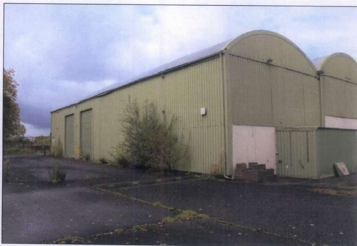
9. The south elevation of the industrial building
