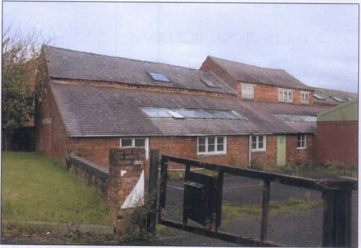
5. The single-storey outrigger at the south end of the west-east range, which is the element attached to the application building, is probably mid-20 th century
