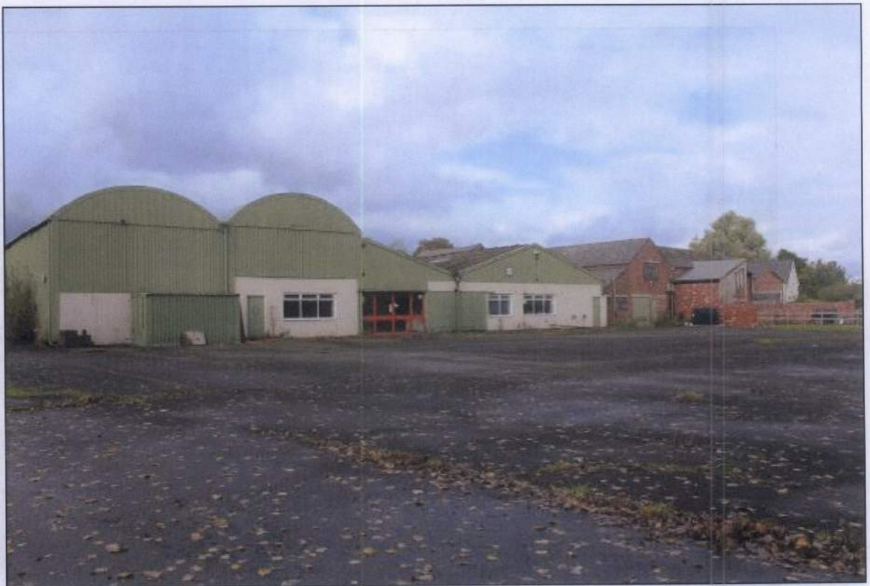
8. Distant view from east showing relationship of the industrial building, the outbuildings and New Holt Lodge Farm beyond
