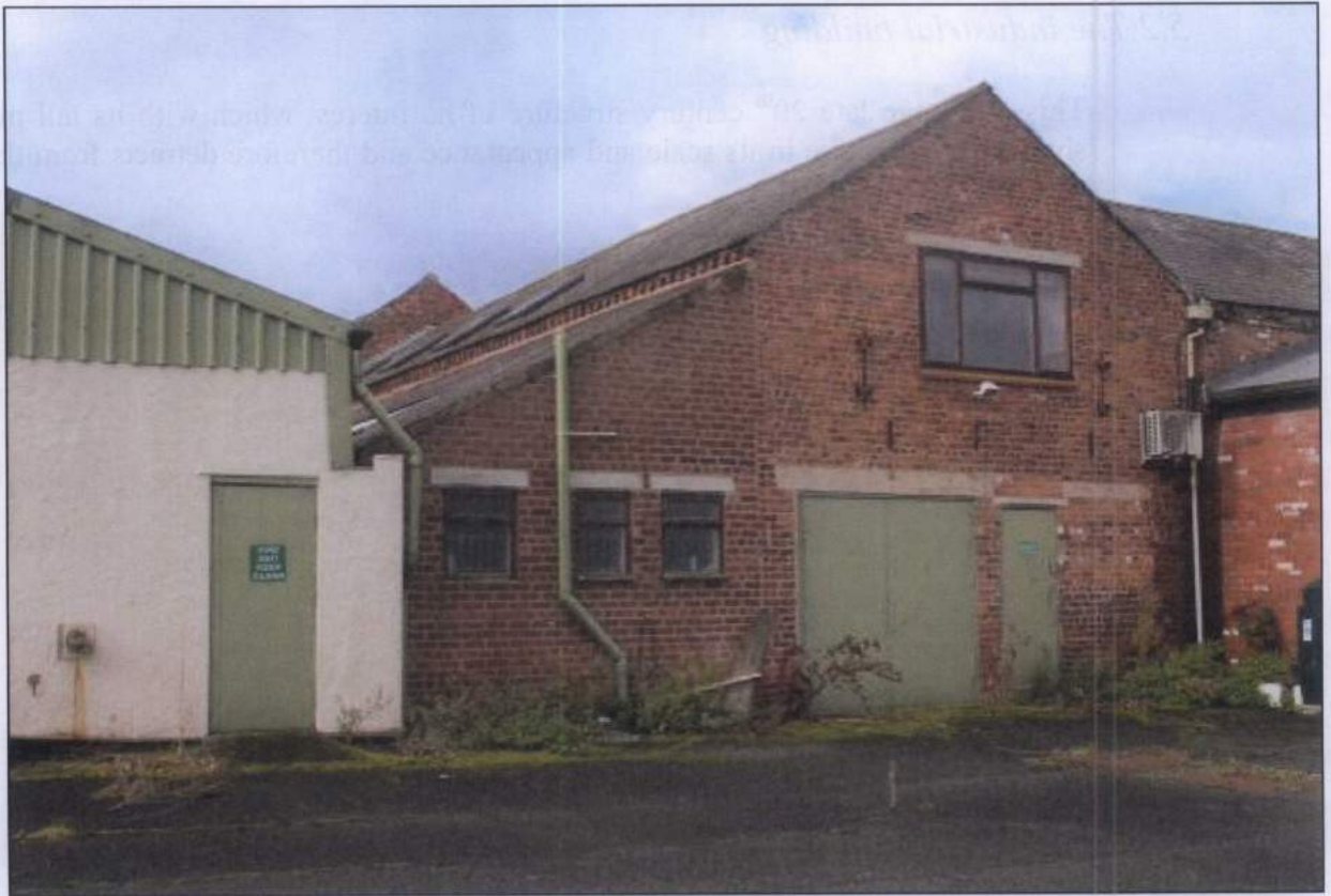
7. East end of the west-east range showing relationship with the industrial building (left)
