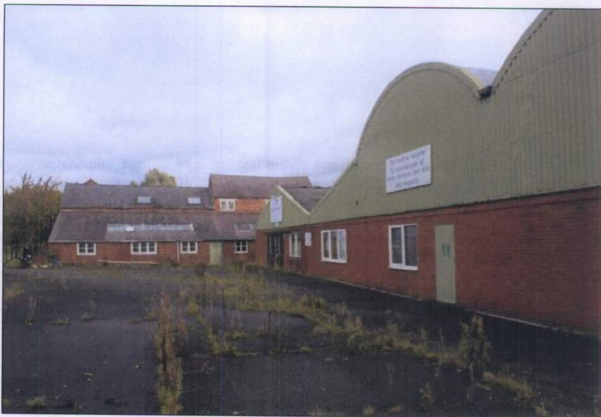
1. The application property, looking north towards the attached outbuilding of New Holt Lodge Farm
