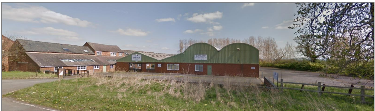
Figure 6 - Image of existing buildings on site
