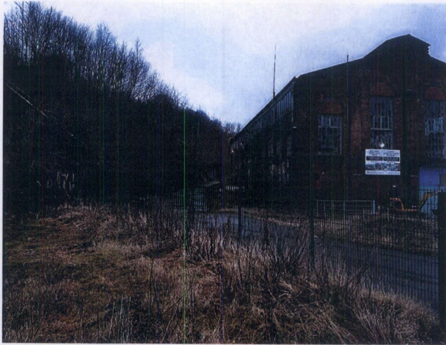
Photograph 3 Southern side of site showing ground level rising rapidly to the south
