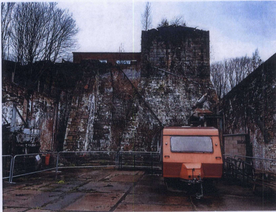
Photograph 9 Steel works structures on site
