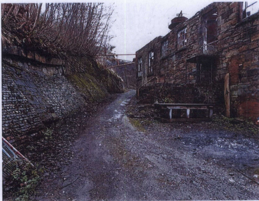
Photograph 13 Same path heading upslope
