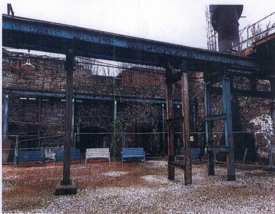
Photograph 8 Adit inside right had entrance
