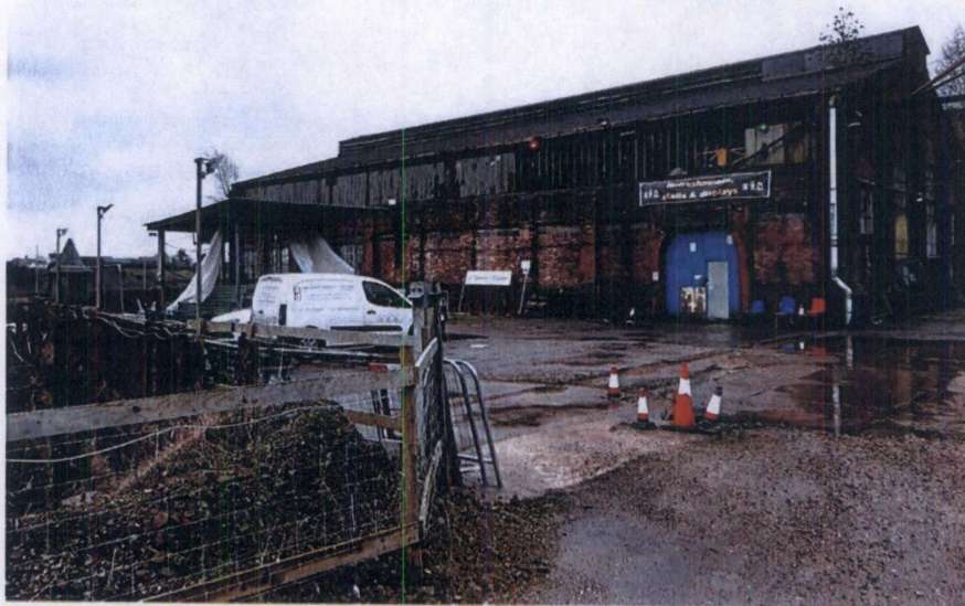
Photograph 4 Main building at front of site
