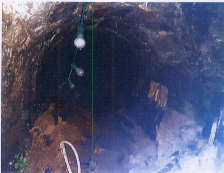
Photograph 11 View up adit
