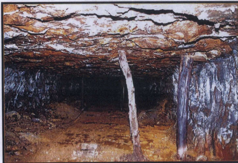
Example of Mine roadway
