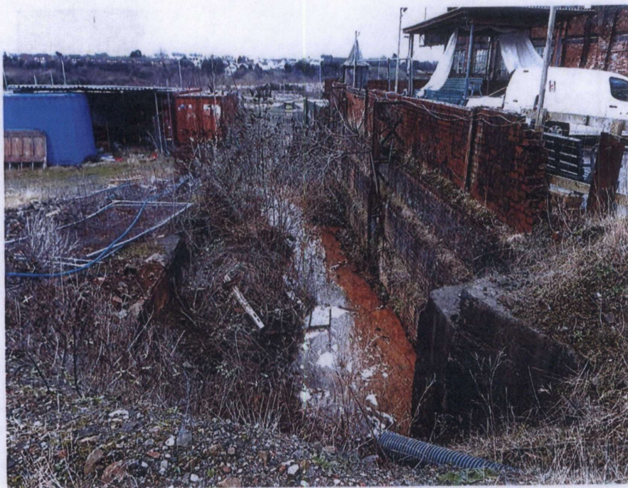
Photograph 5 drainage channel through site
