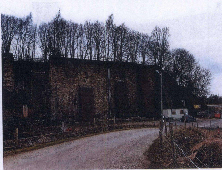
Photograph 6 Retaining structure on northern site boundary
