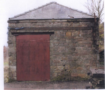
Timber boarded double doors to be reinstated as image on existing photographic record sheet SK06. Framed, vertically boarded, T&G square edged doors
