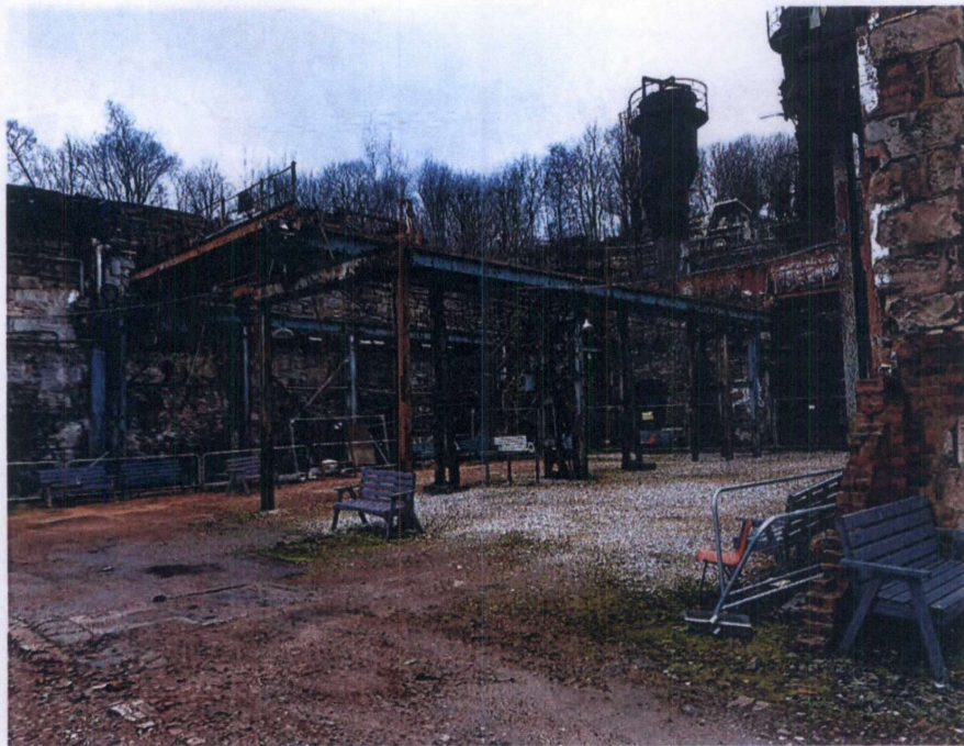
Photograph 7 Inside previous building
