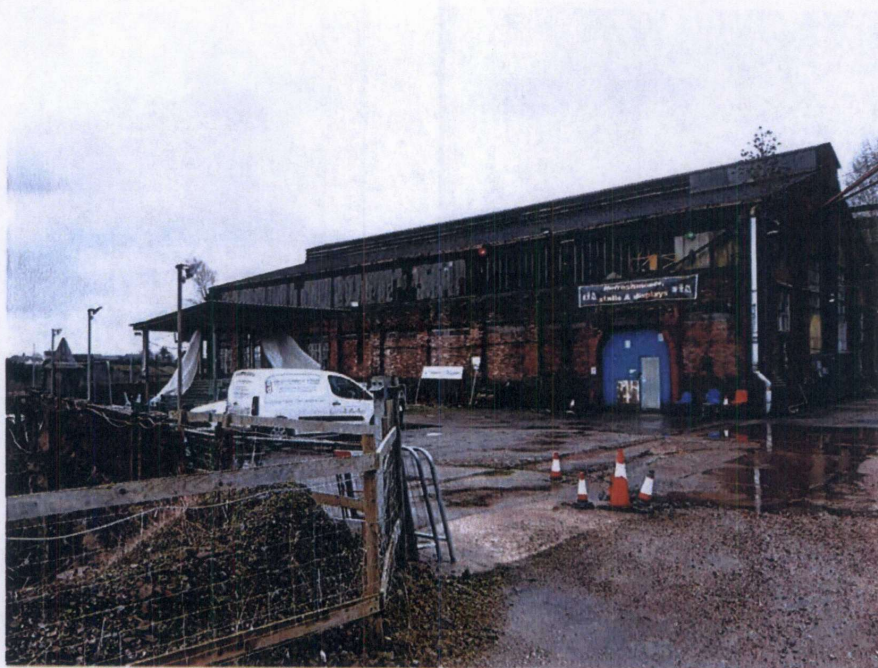
Photograph 4 Main building at front of site
