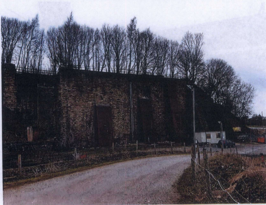
Photograph 6 Retaining structure on northern site boundary
