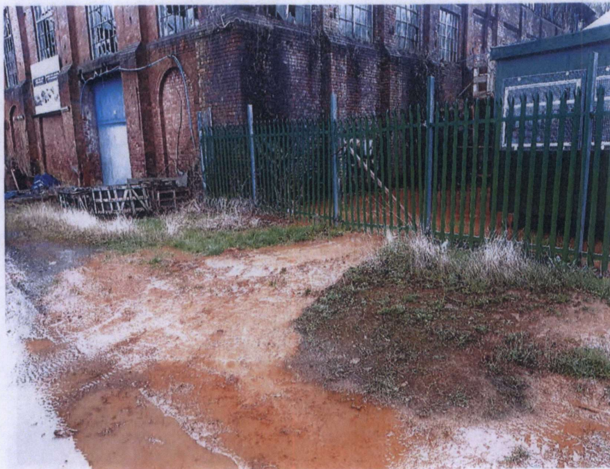
Photograph 1 Mine water discharge from adit
