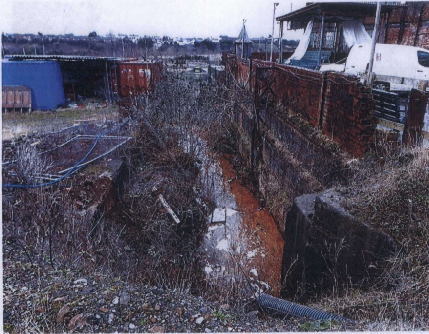
Photograph 5 drainage channel through site
