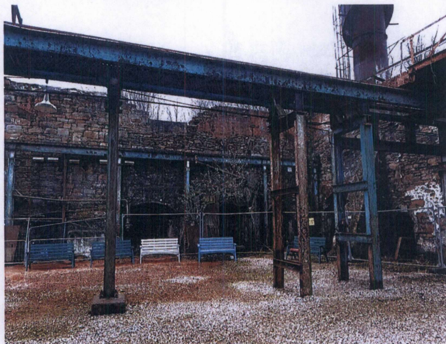
Photograph 8 Adit inside right had entrance
