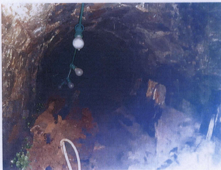
Photograph 10 View up adit
