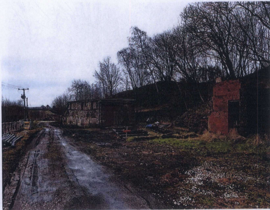
Photograph 13 Agents house, which is on the old plans
