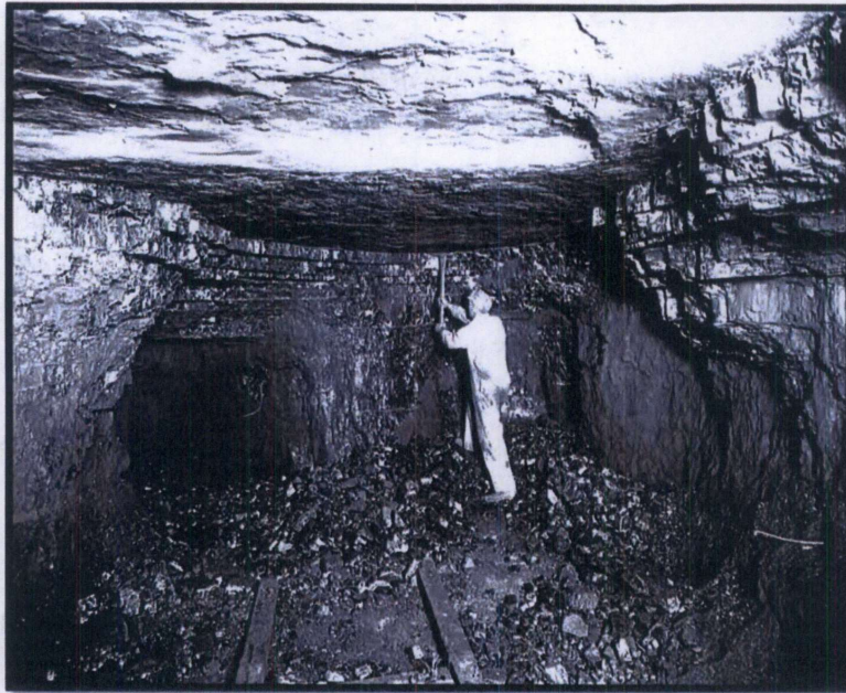
Coal being works with pillars either side
