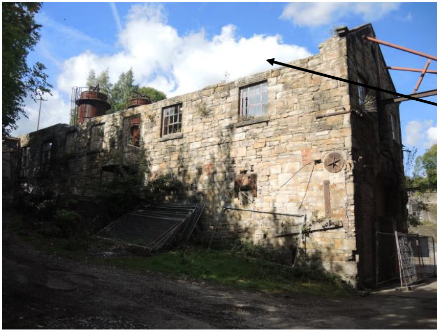
Timber windows to be carefully removed and like for like repairs undertaken, piecing in new timber when necessary
