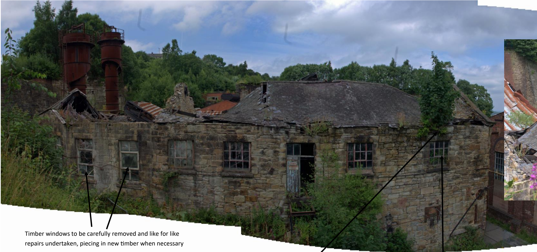
Metal windows to be deglazed, removed and overhauled before being refixed on a like for like basis
