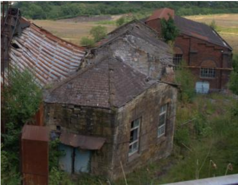
Between 4-5 additional courses of stonework need to be rebuilt over the head of the existing windows to realign with the gable and the rest of the elevation
