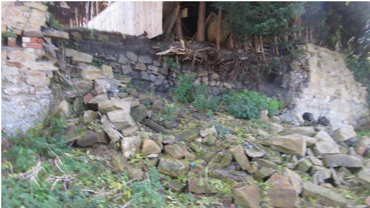
Image 3.9 internal wall collapse
