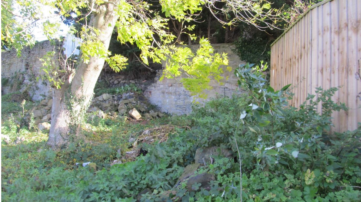
Image 3.9 internal wall collapse
