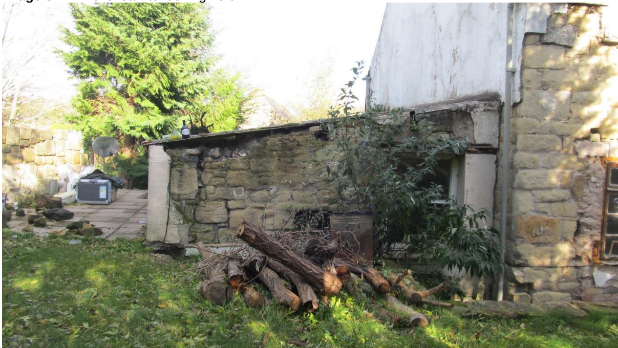
Image 3.4 B1 the lean-to looking north
