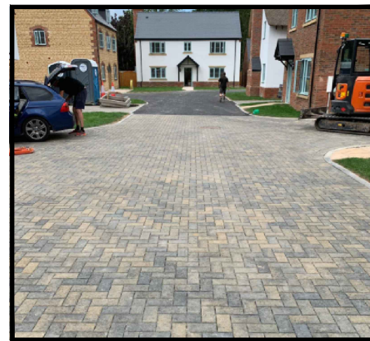
Permeable Block paving
