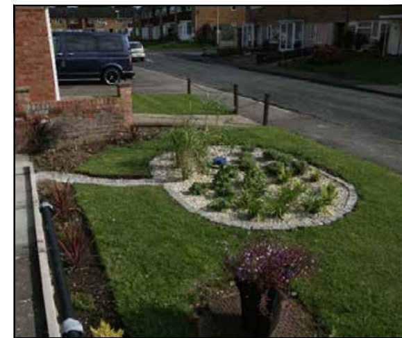
SUDS Rain Garden
