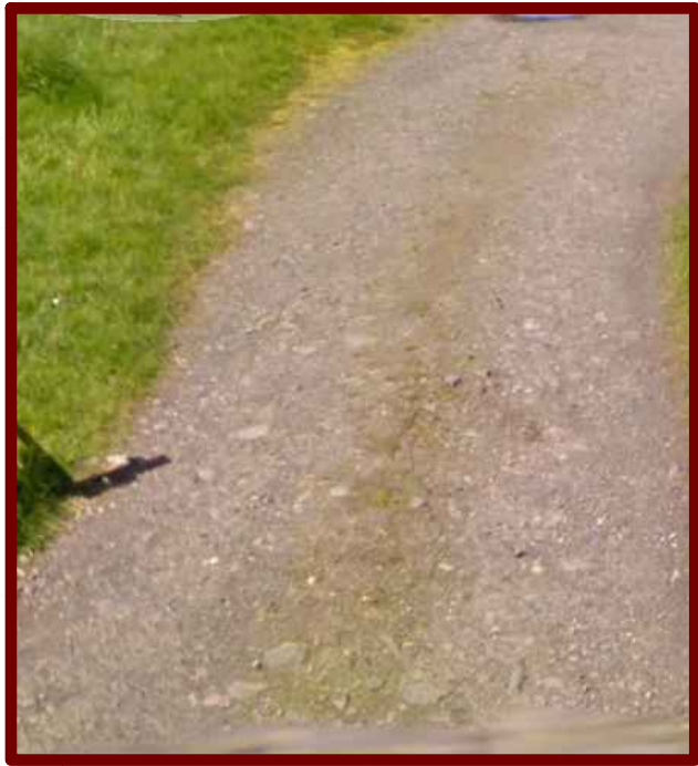
Existing Track Road
