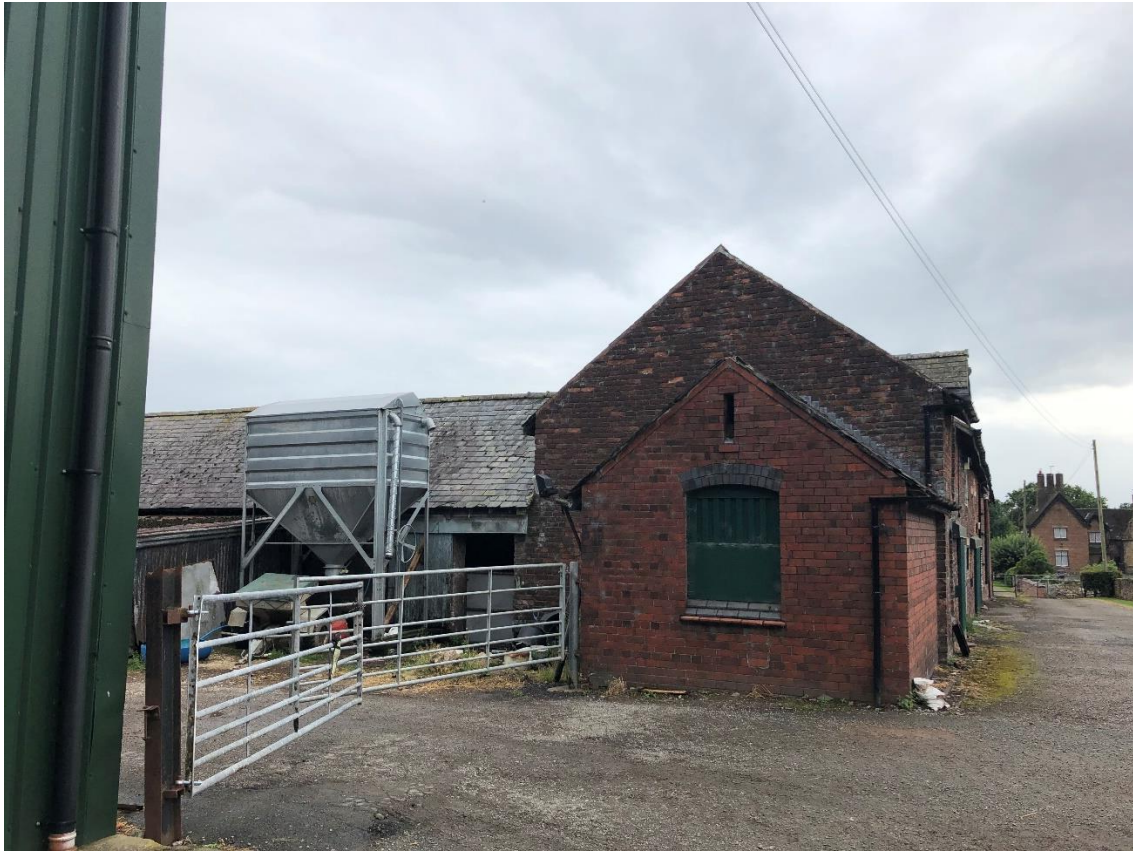
PLATE 5 YARD AREAS AND FARMHOUSE IN BACKGROUND
