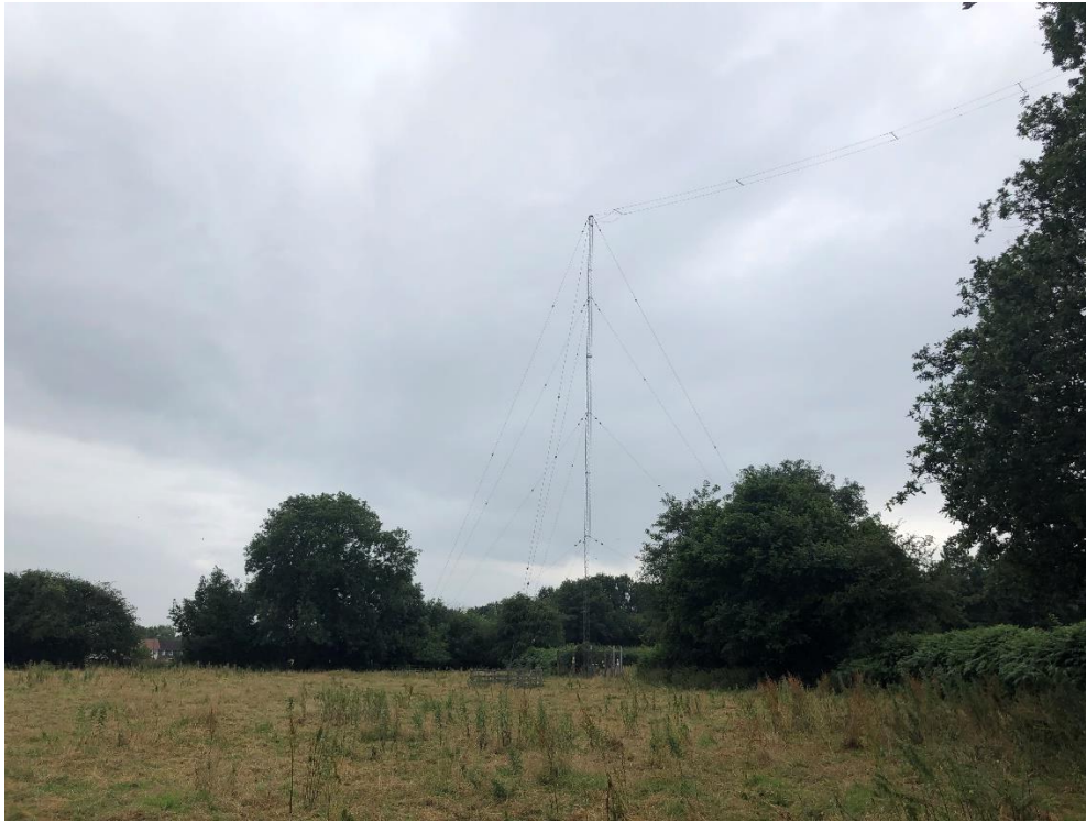
PLATE 3 – GENERAL SURFACE CONDITIONS IN THE SOUTH OF THE SITE AND MAST IN BACKGROUND
