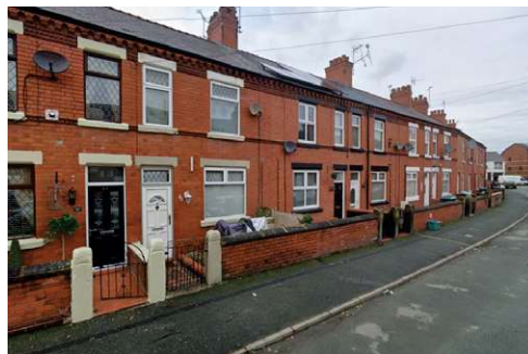
Terraced properties along Edward Street
