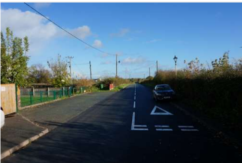
20. View along Bersham Lane and southern boundary of site
