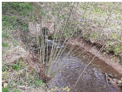
Figure 24: Concrete culvert where TN2 water emerges from under Berse Lane
