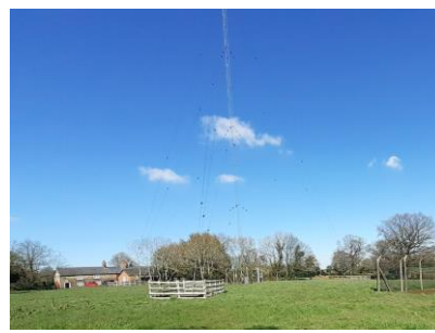
Figure 35: Large mast in the field near TN26
