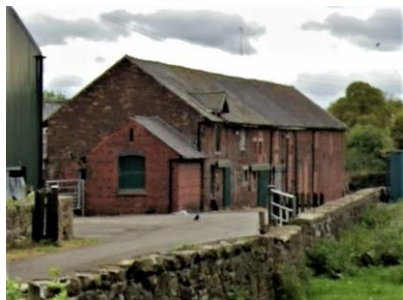
Figure 32: Old brick multipurpose farm building
