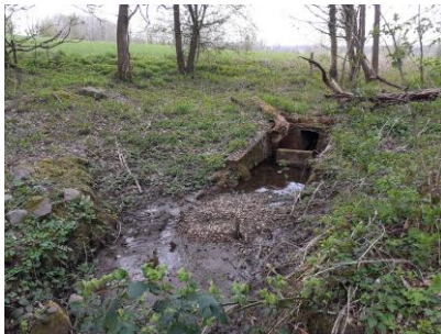
Figure 30: Outfall of TN25 culvert into the woodland of TN9
