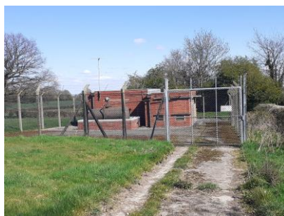
Figure 34: Electricity sub-station at TN28
