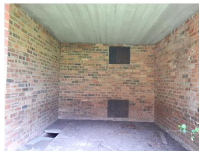
Figure 39: Inside of the small brick building at TN23
