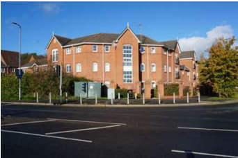
Flats along Ruthin Road
