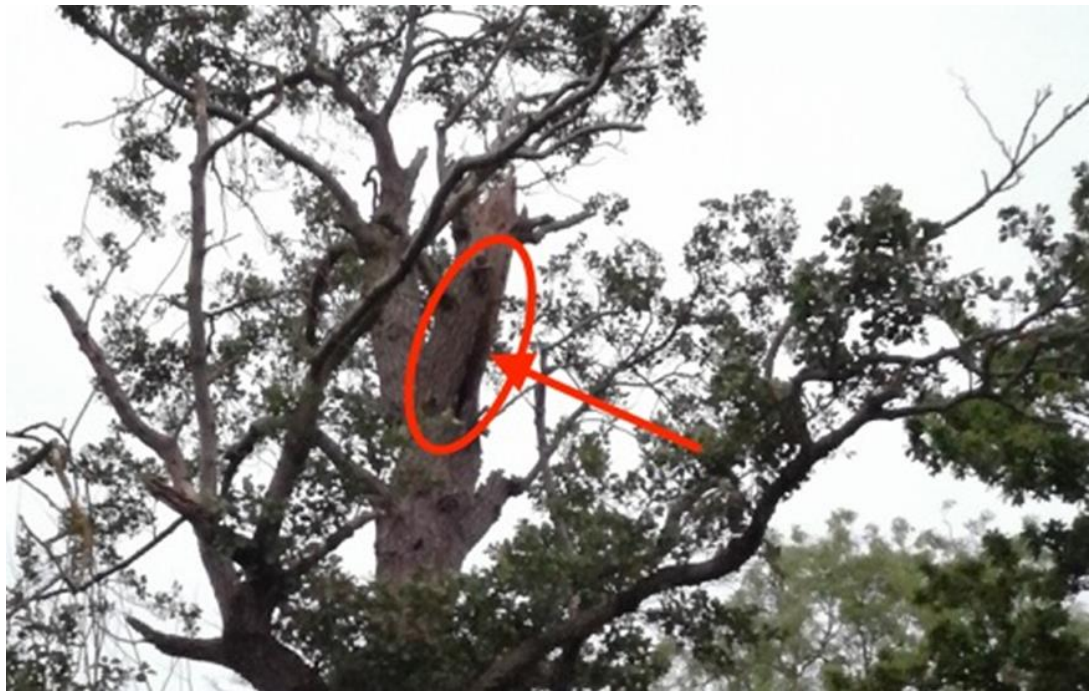
Figure 18. Trunk cavity on north-west aspect of alder tree T172.
