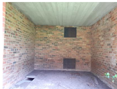
Figure 39: Inside of the small brick building at TN23
