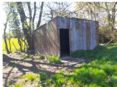
Figure 33: Corrugated metal field shelter at TN27
