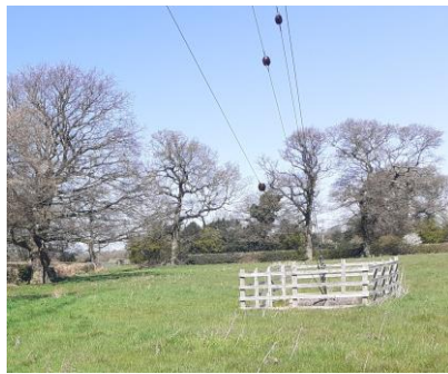
Figure 36: Stabilising anchor points for the large mast
