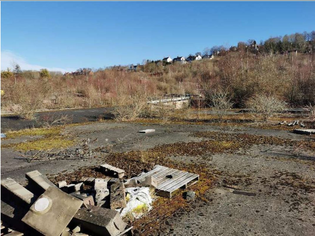
Plate 26. – Hardstanding surfacing and overgrown vegetation. Localised fly tipping.
