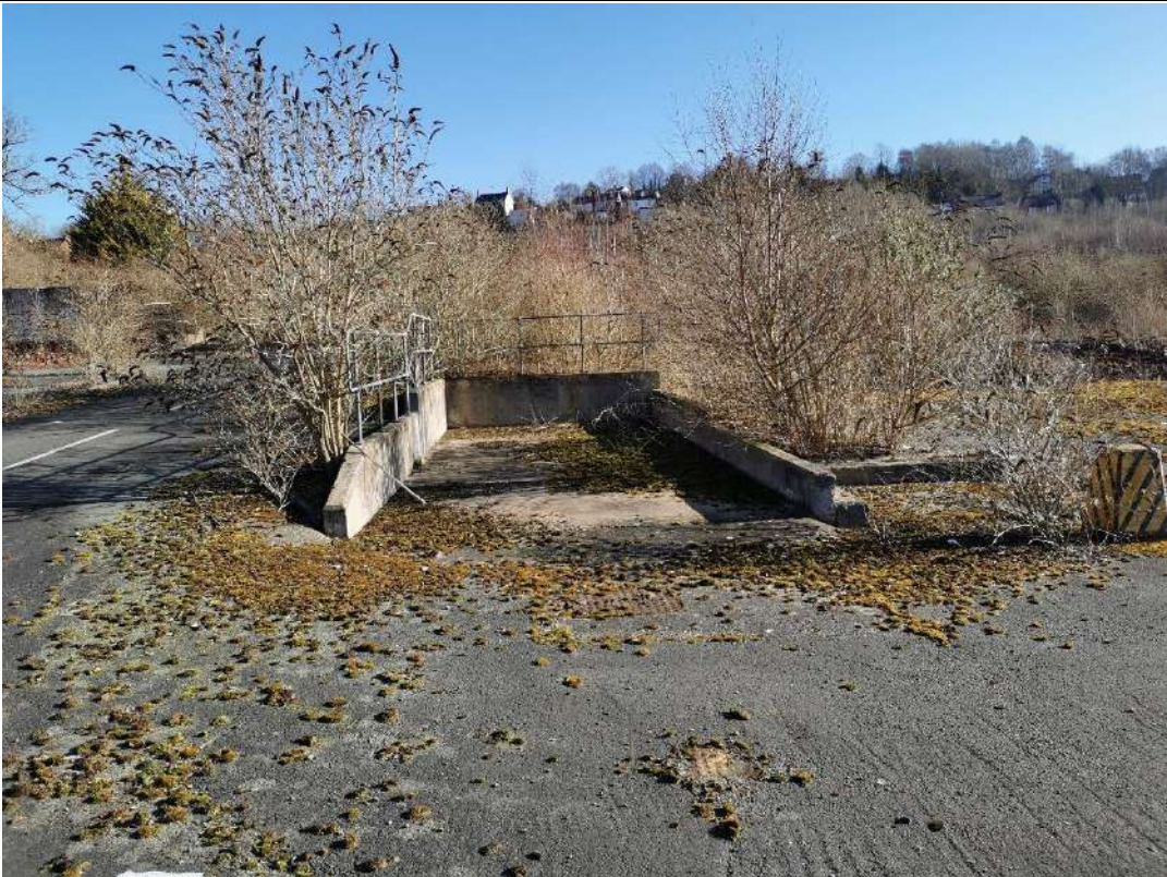
Plate 10. – Hardstanding surfacing and overgrown vegetation. Evidence of historic industrial features
