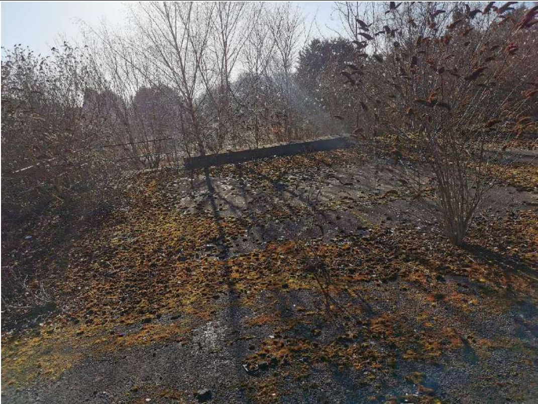
Plate 18. – Hardstanding surfacing and overgrown vegetation. Evidence of historic industrial features
