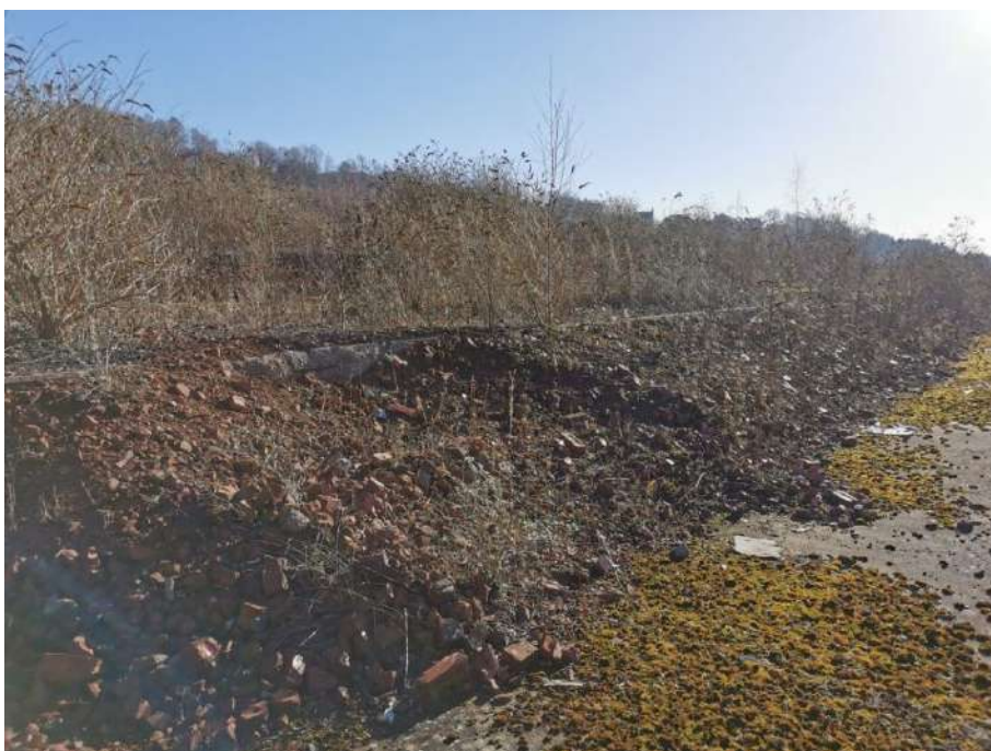
Plate 3: Demolition rubble in north-western part of Site
