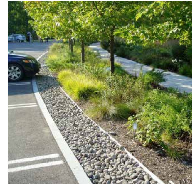
Figure 03-4: SuDS and drainage
