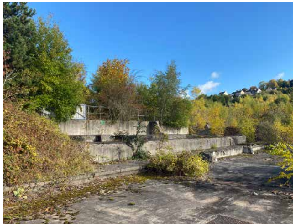
Figure 11. View C Remnant of the former industrial use. Existing reinforced concrete slabs and retaining walls
