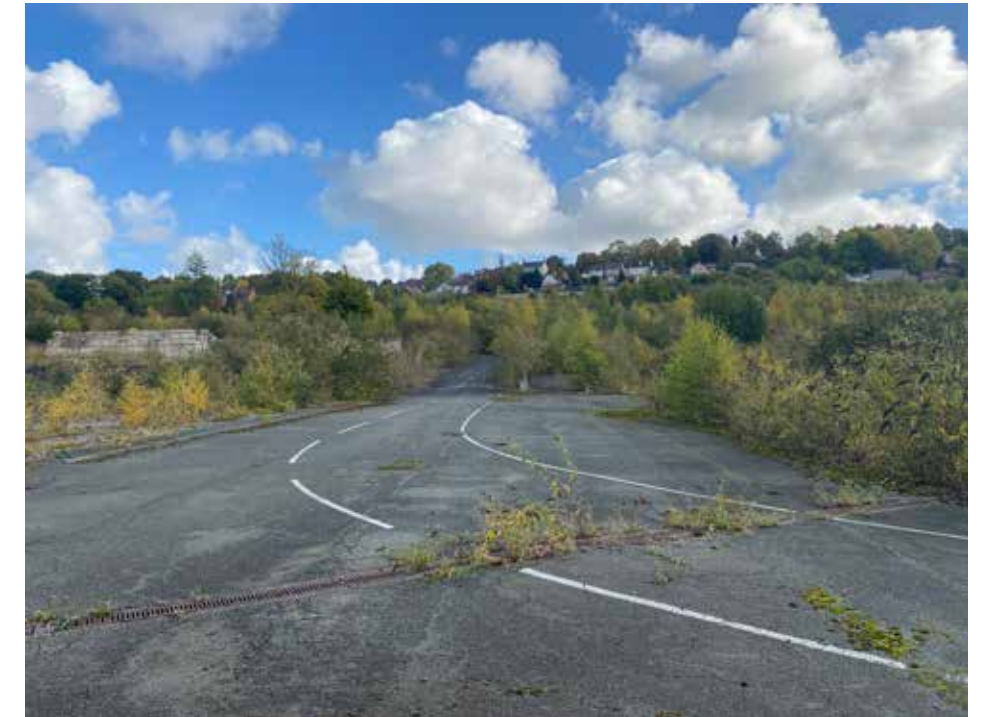
Figure 10. View B west from within the centre of the site. Concrete foundations at base level, with Buddleja growing within gaps.
