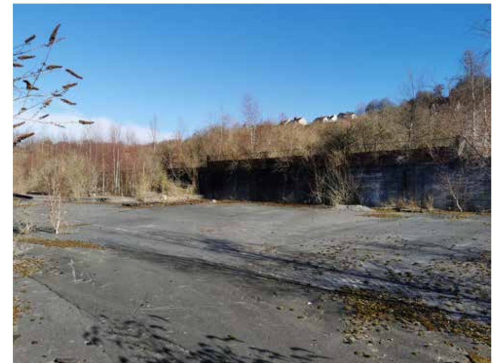
Figure 12. View D looking north showing existing brick retaining wall and concrete building foundations
