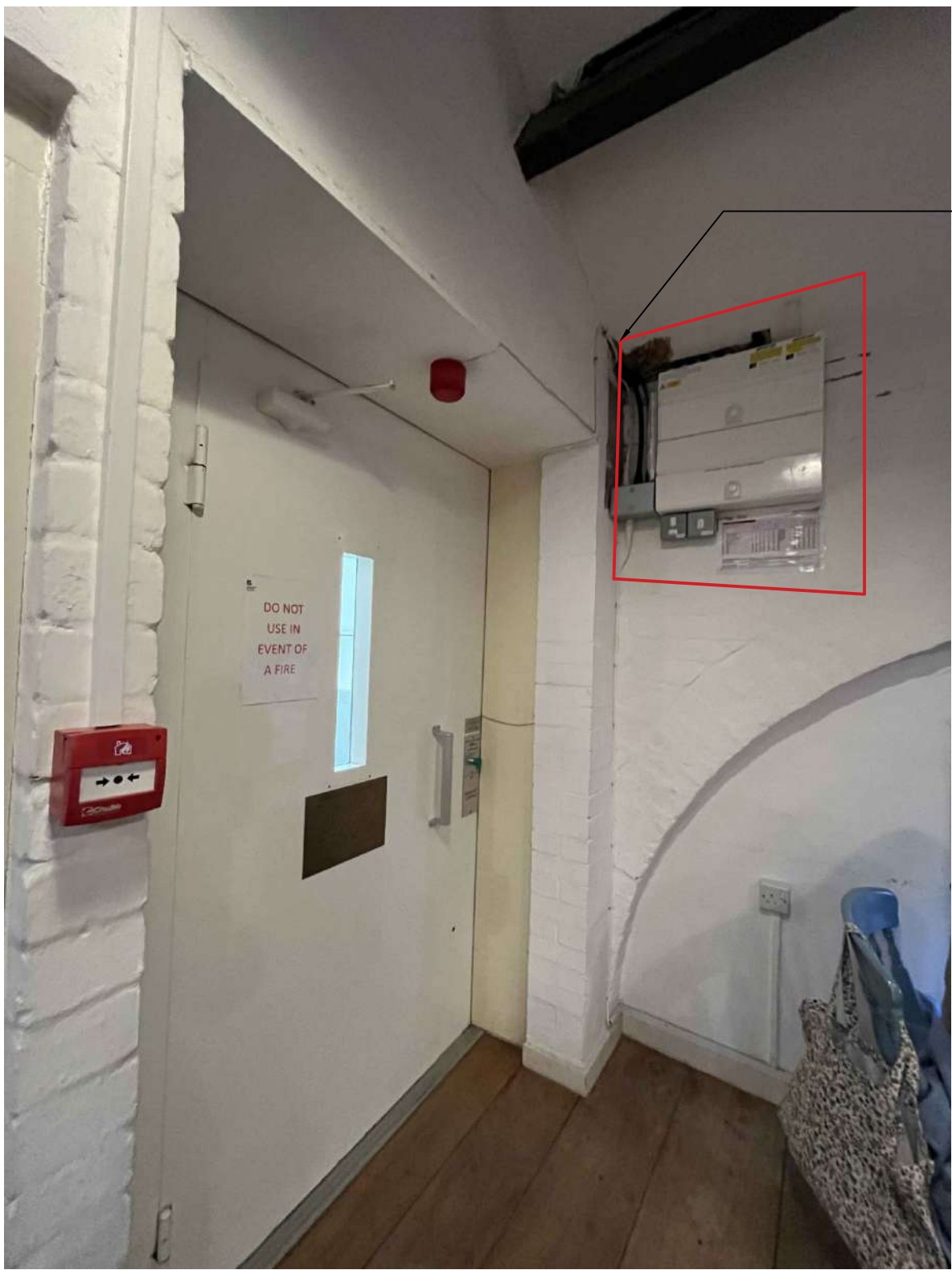
Image 01 Electrical box viewed from inside the Restaurant to be boxed up as it is above emergency escape route
