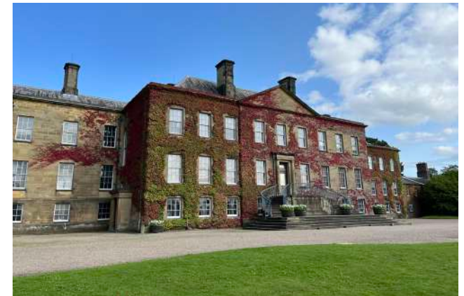
Present day image of the rear elevation
