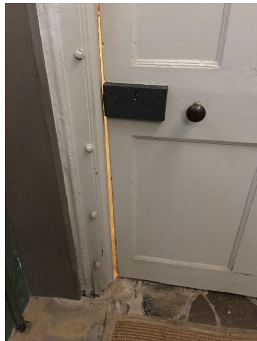
Closed door G22 showing warping
