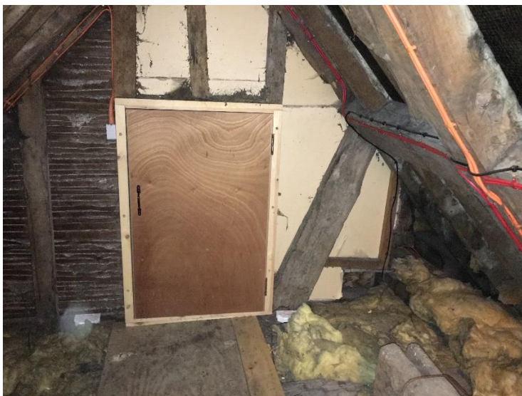
Barrier D lath and plaster
