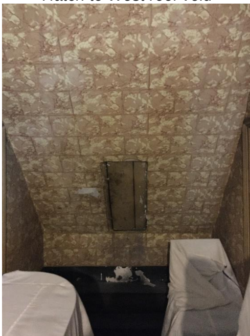
Hatch to West roof void
