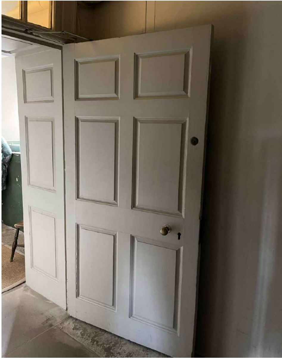
Image 3 - Precedent panelled door for dimensions - Door 20 - Ground Floor main house - between G19 & G17 Fanlight above this door also used as precedent for glazing..
