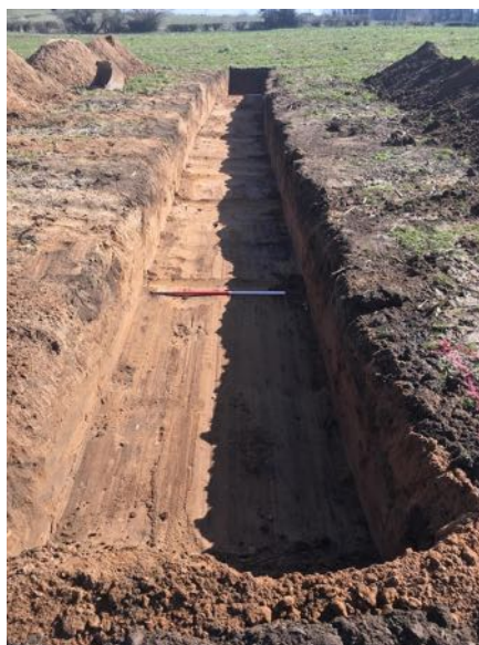
Plate 16- Overview of Trench 9. Facing east, 1m scale.
