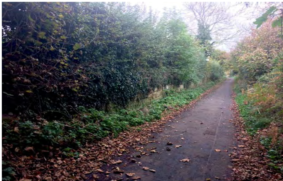
Plate 7: East facing view along Bryn Estyn Road. The revetting wall (82626) can be seen on the left side
