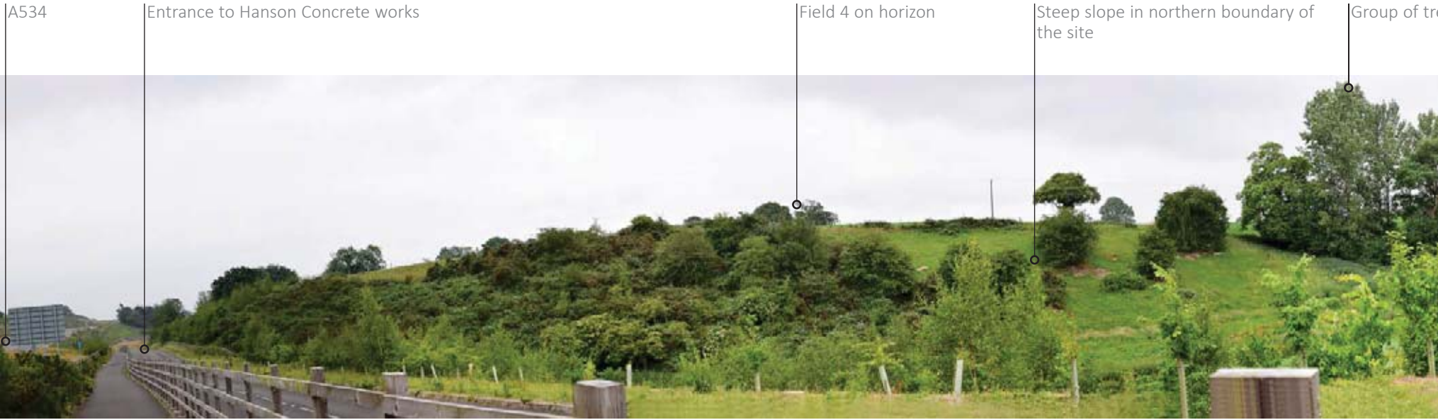
Photo 1.5 - View from the footpath along the A534 looking east.
