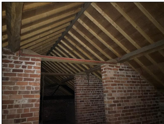
Plate 6. First floor of western end of Barn
