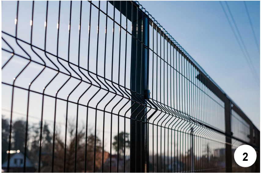
BOUNDARY SECURITY FENCE 2.4m High Paladin Fence
