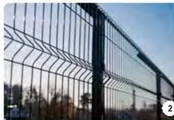
BOUNDARY SECURITY FENCE 2.4m High Paladin Fence
