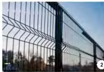
BOUNDARY SECURITY FENCE 2.4m High Palatin Fence
