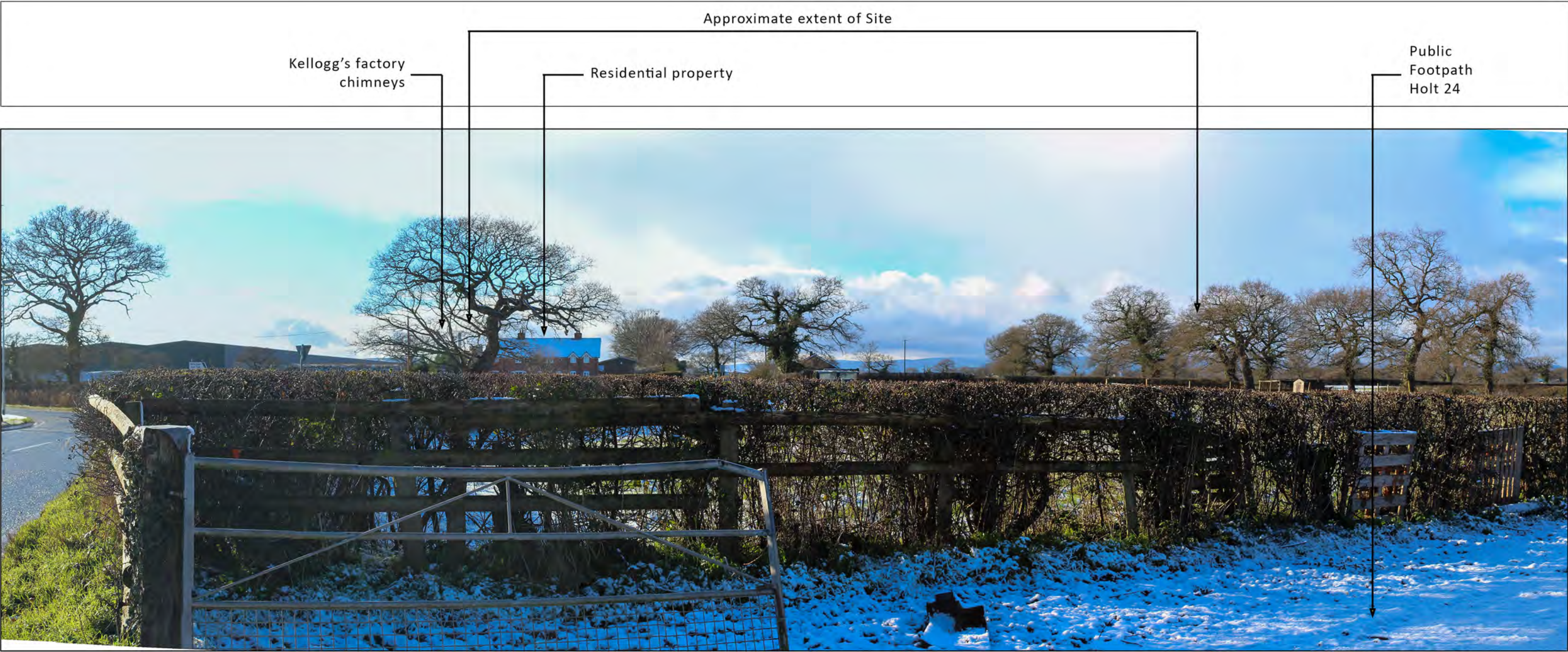
Location: Public Footpath Holt 24, looking west towards the Site.
