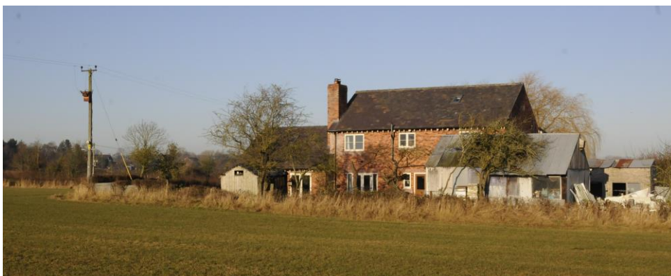
Figure 10 View of the south side of Honeysuckle Cottage (NDHA88), looking north
