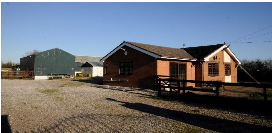
Figure 34 The modern buildings at the east side of Field 8
