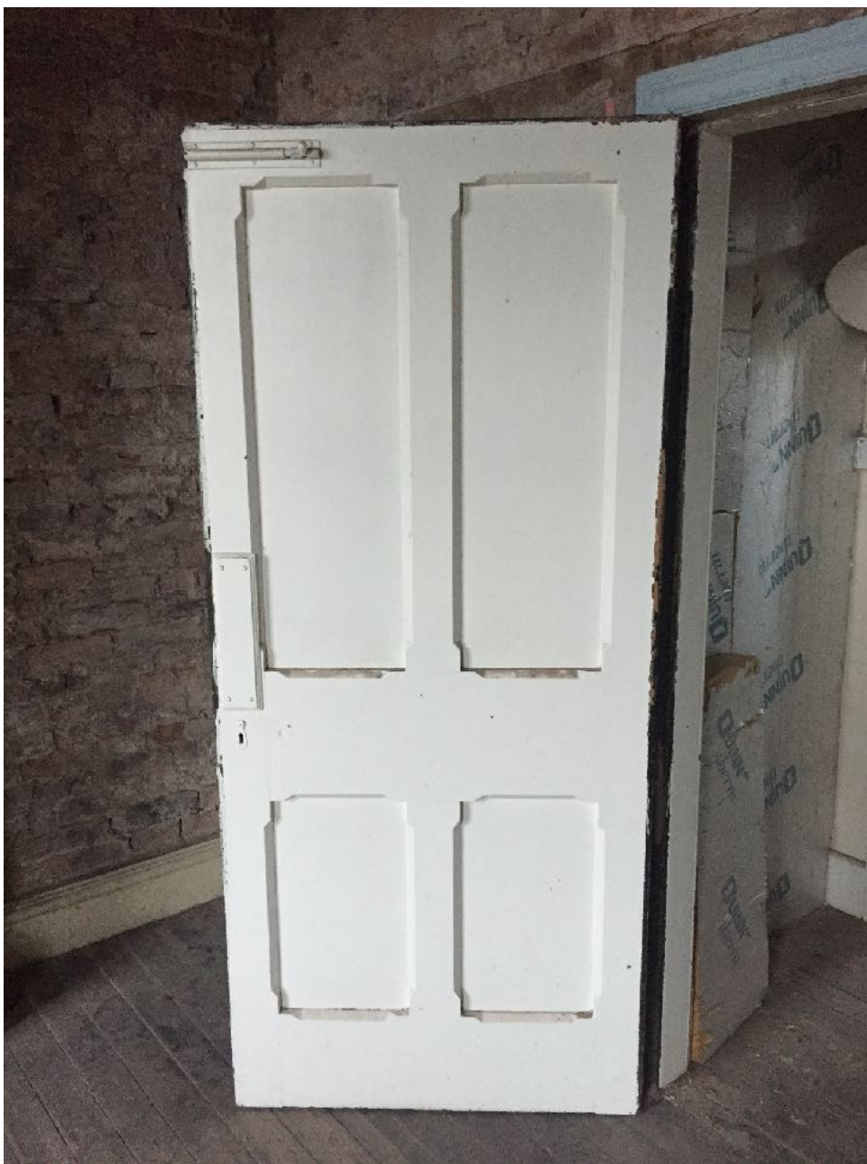
Victorian 4-panelled door.
