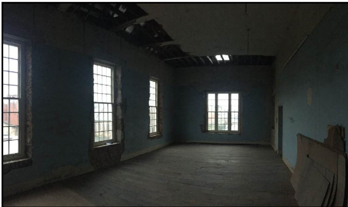
First Floor Apartment 3 (Green) facing south
