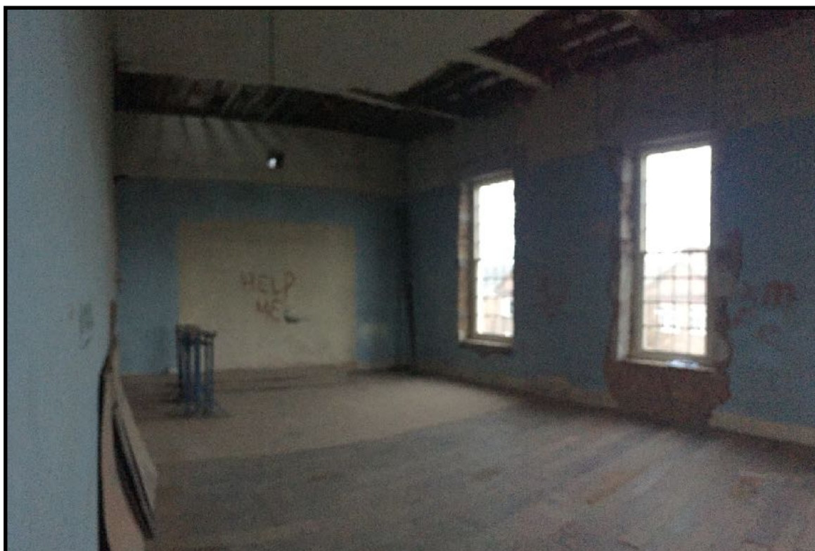
First Floor Apartment No. 3 (Green) facing north towards blocked up opening in rear elevation. A pair of windows is proposed for this elevation as shown in the drawings.
