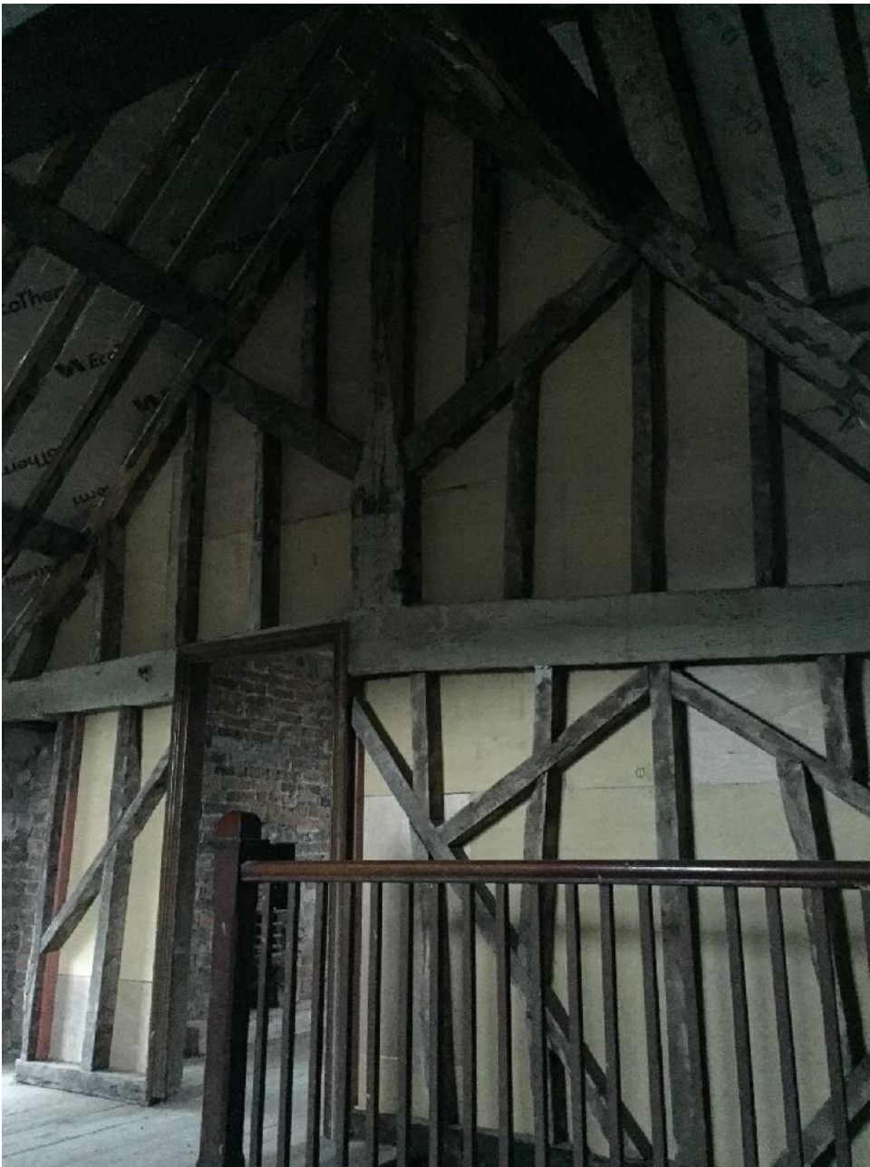
Victorian style Y-shaped truss to internal partition between Room numbers 6 & 7.
