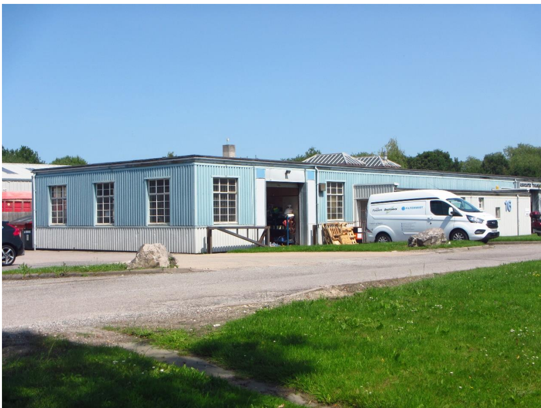
Photograph 20 – Southern and eastern aspect of Building 5.
