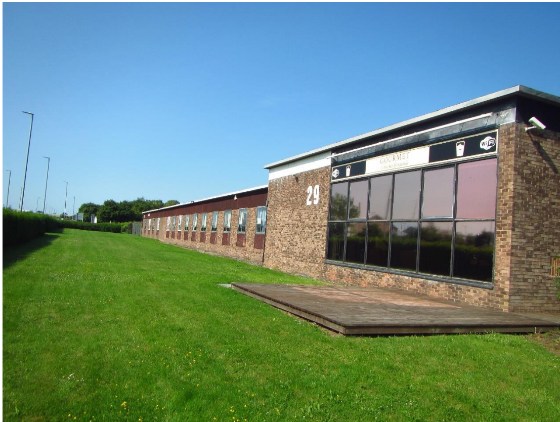
Photograph 1 – Eastern aspect of Building 1.
