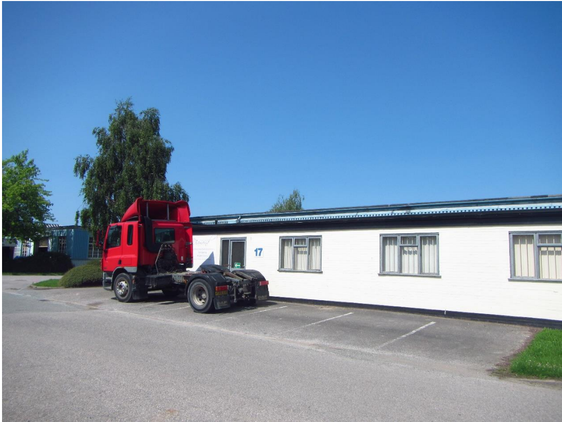
Photograph 19 – Eastern aspect of Building 4.
