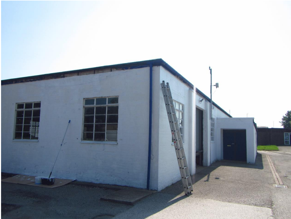
Photograph 11 – Western and southern aspect of Building 2.
