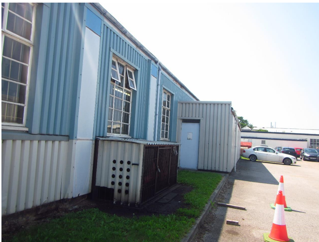
Photograph 21 – Western aspect of Building 5.
