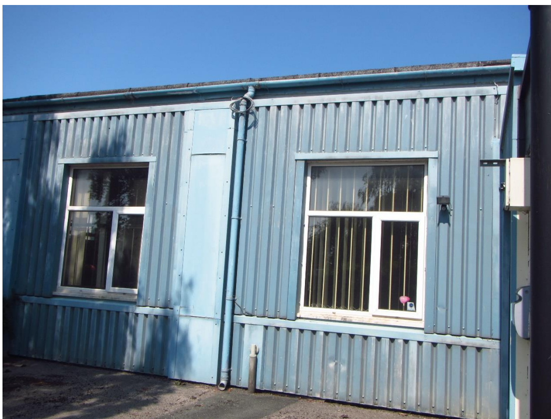
Photograph 14 – Eastern aspect of Building 4.
