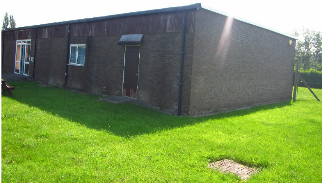
Photograph 2 – Southern aspect of Building 1.
