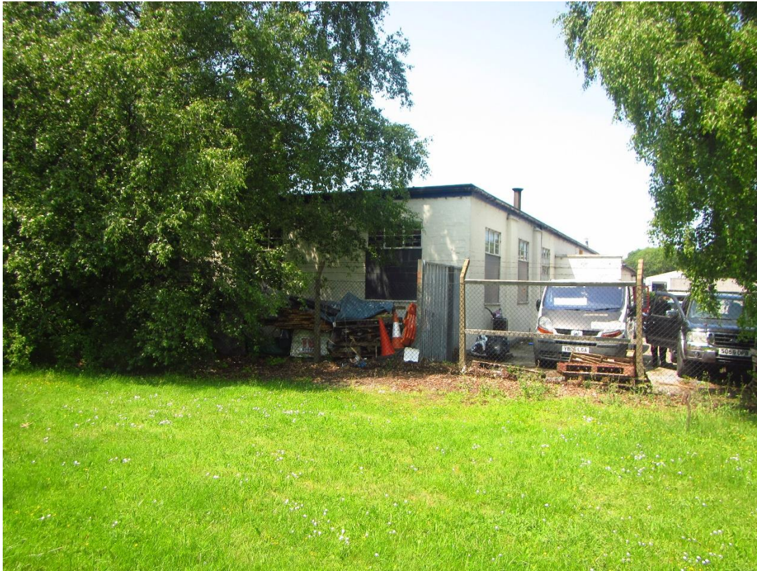
Photograph 23 – Eastern aspect of Building 8.
