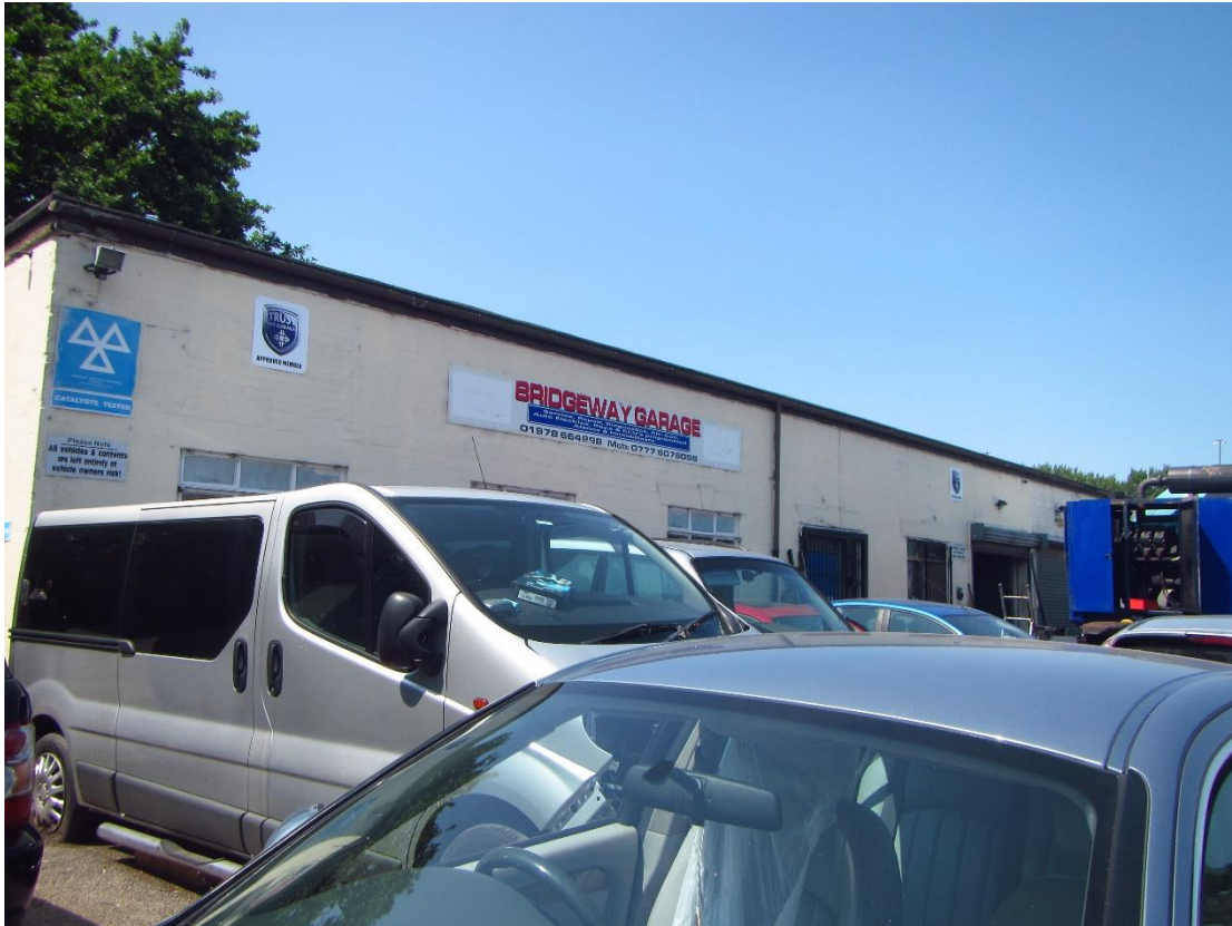
Photograph 24 – Northern aspect of Building 9.
