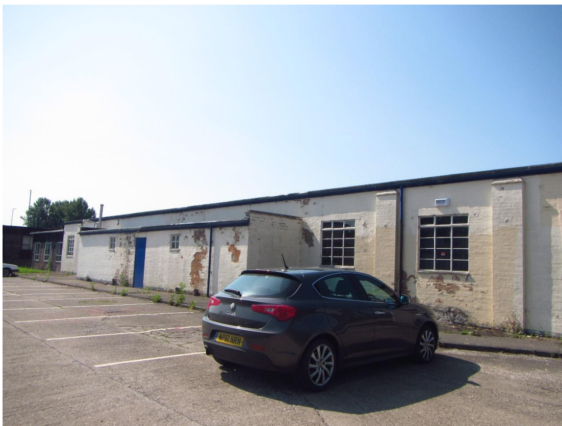
Photograph 7 – Northern aspect of Building 2.
