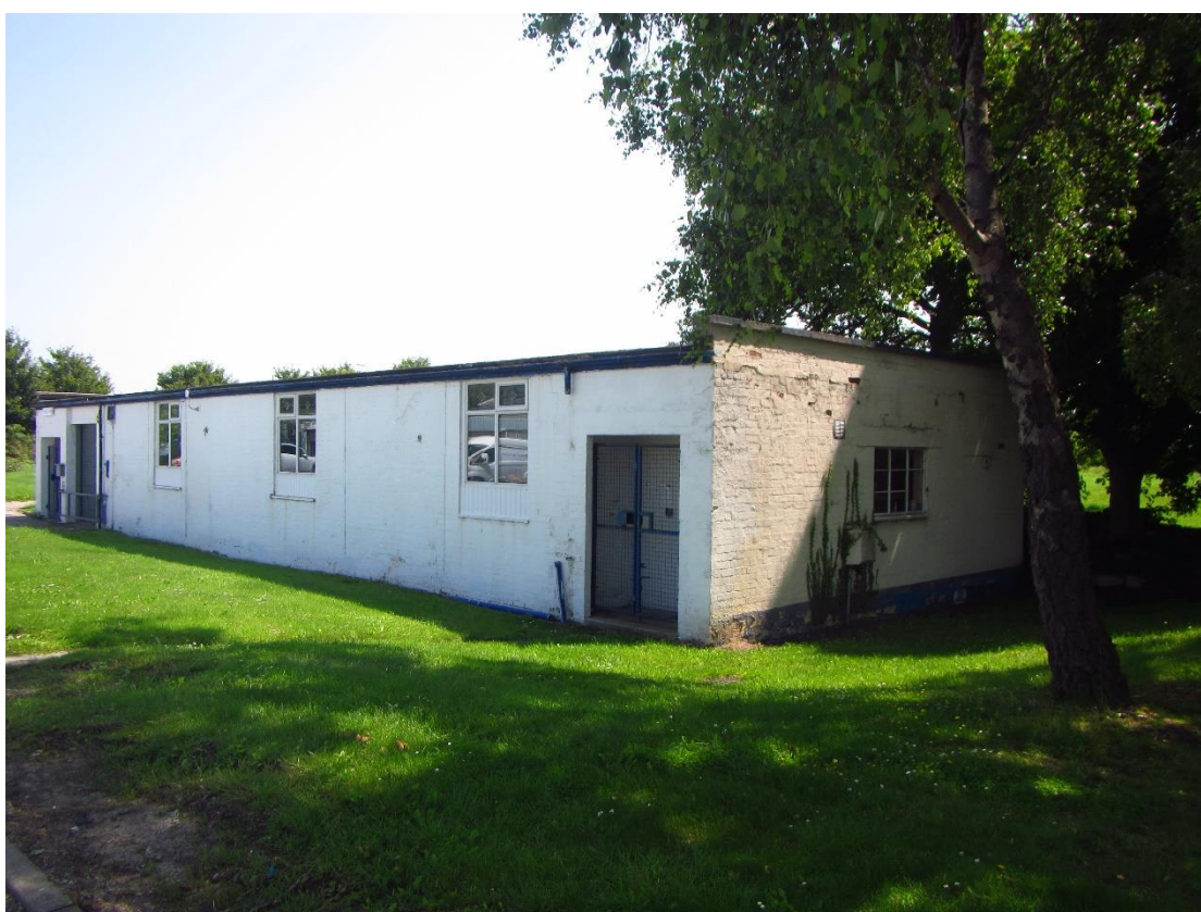
Photograph 22 - Southern and western aspect of Building 6.
