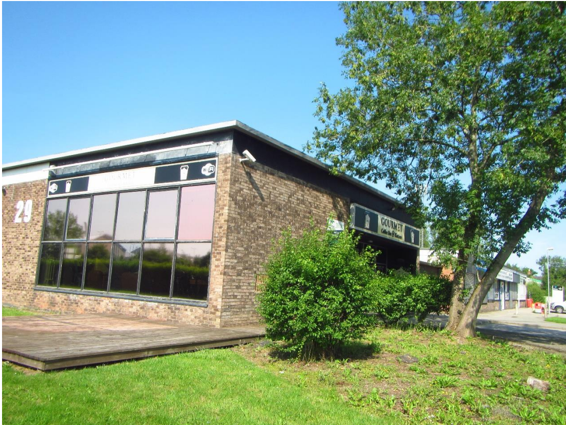
Photograph 6 – Northern aspect of Building 1.
