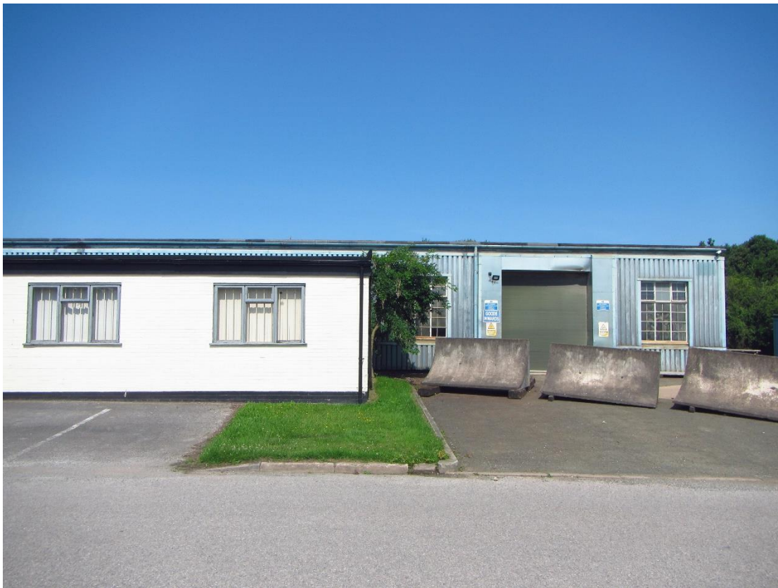
Photograph 18 – Eastern aspect of Building 4.
