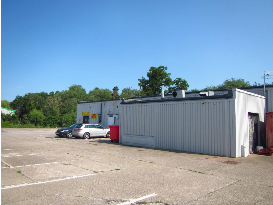
Photograph 5 – Southern aspect of Building 1.
