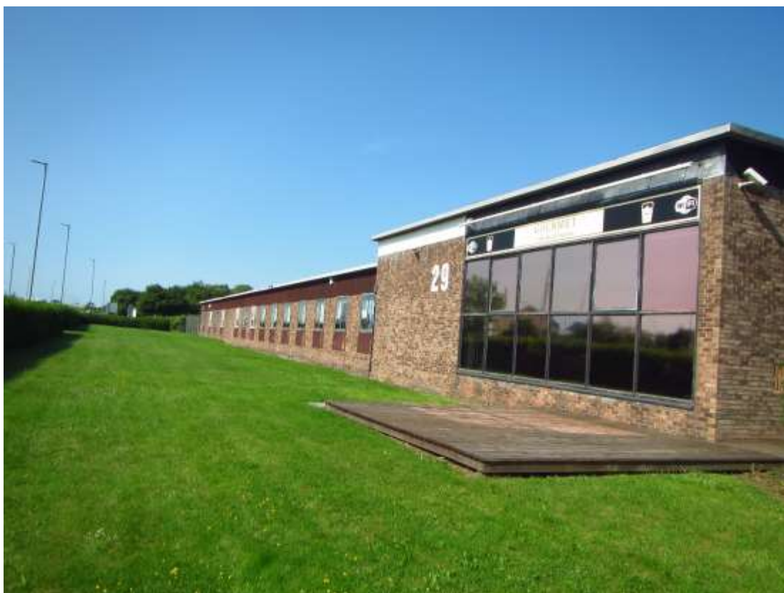
Photograph 1 – Building 1, adjacent to the eastern site boundary.
