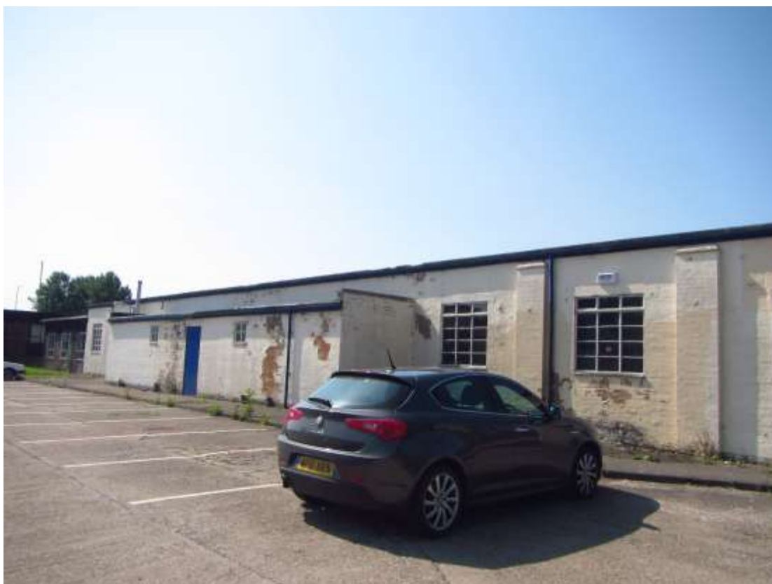
Photograph 7 – Northern aspect of Building 2.
