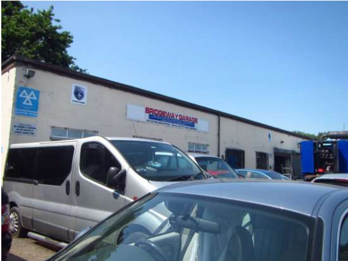
Photograph 24 – Northern aspect of Building 9.
