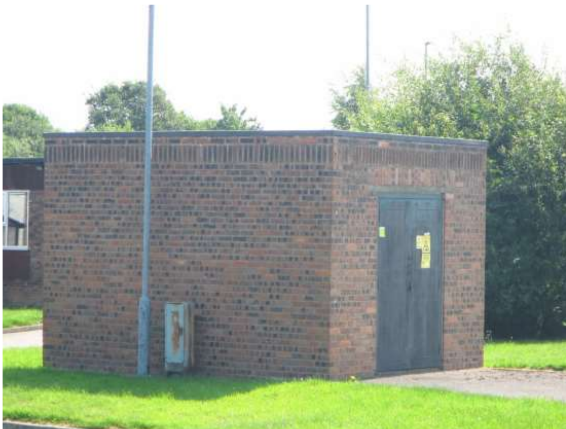
Photograph 25 – Western and southern aspect of Building 10.
