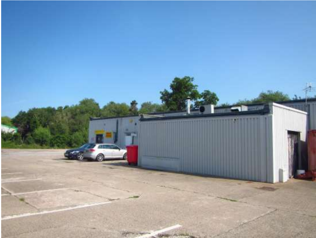
Photograph 5 – Southern aspect of Building 1.
