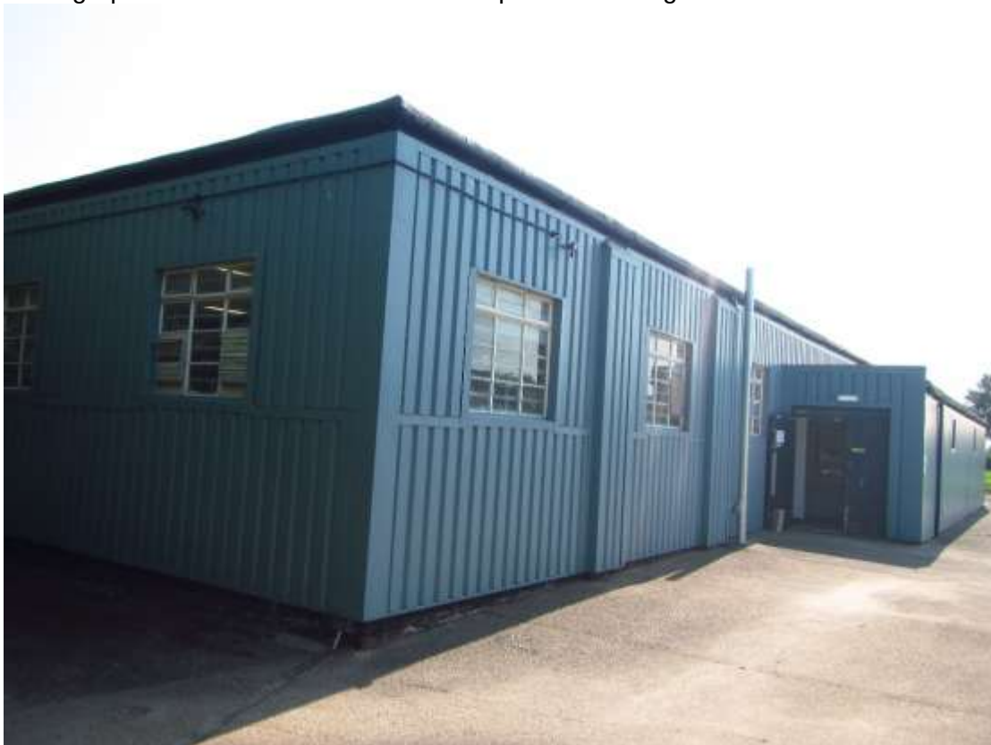
Photograph 12 – Western and southern aspect of Building 3.
