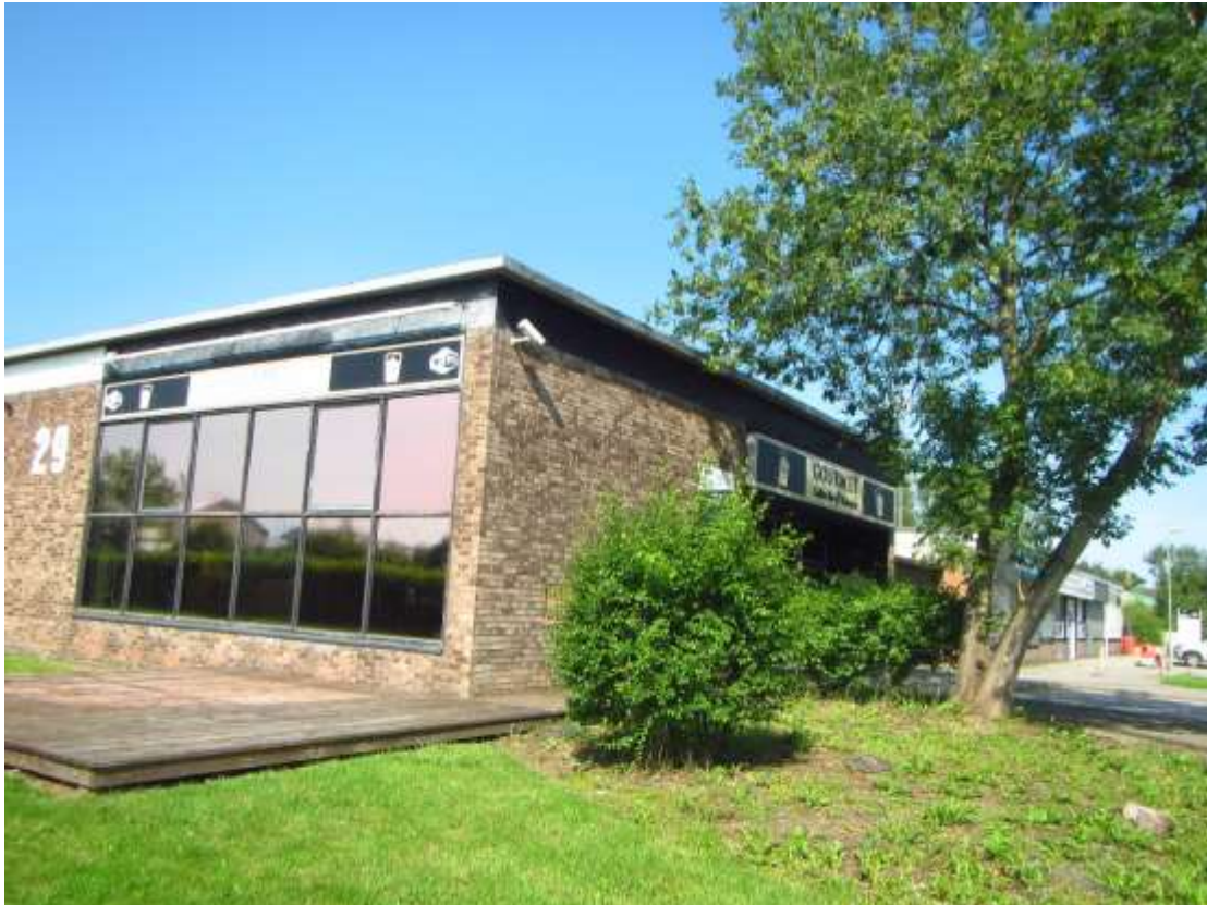
Photograph 6 – Northern aspect of Building 1.
