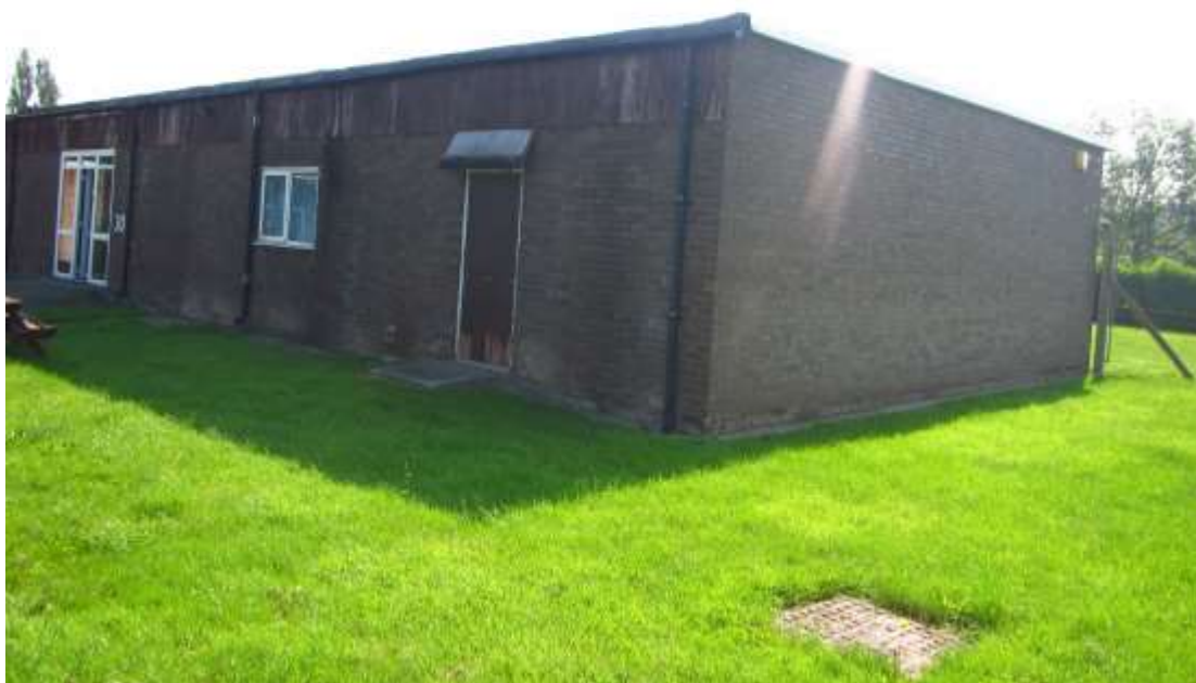
Photograph 2 – Southern aspect of Building 1.
