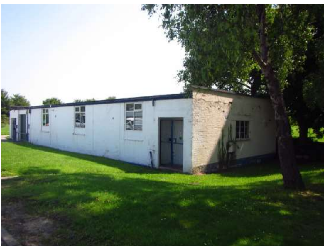
Photograph 22 - Southern and western aspect of Building 6.
