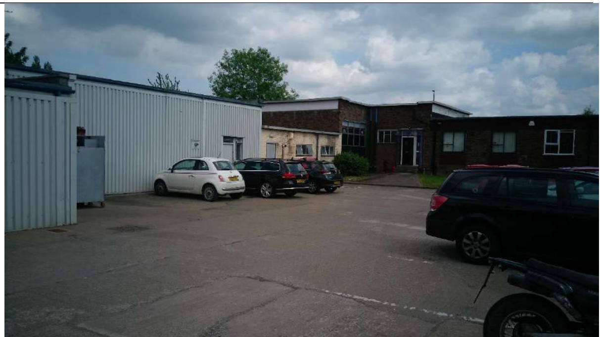
Plate 2: The Bridgeway Centre
