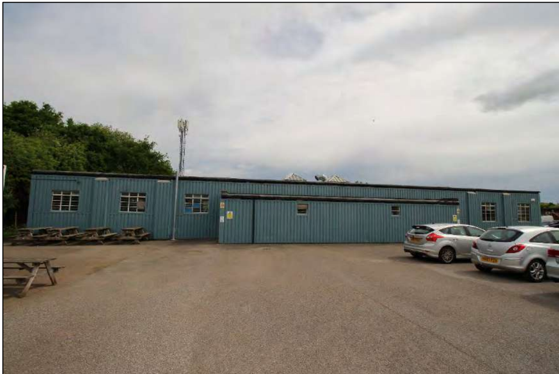
Plate 35: Rear south-west elevation of Building 3, looking north-east
