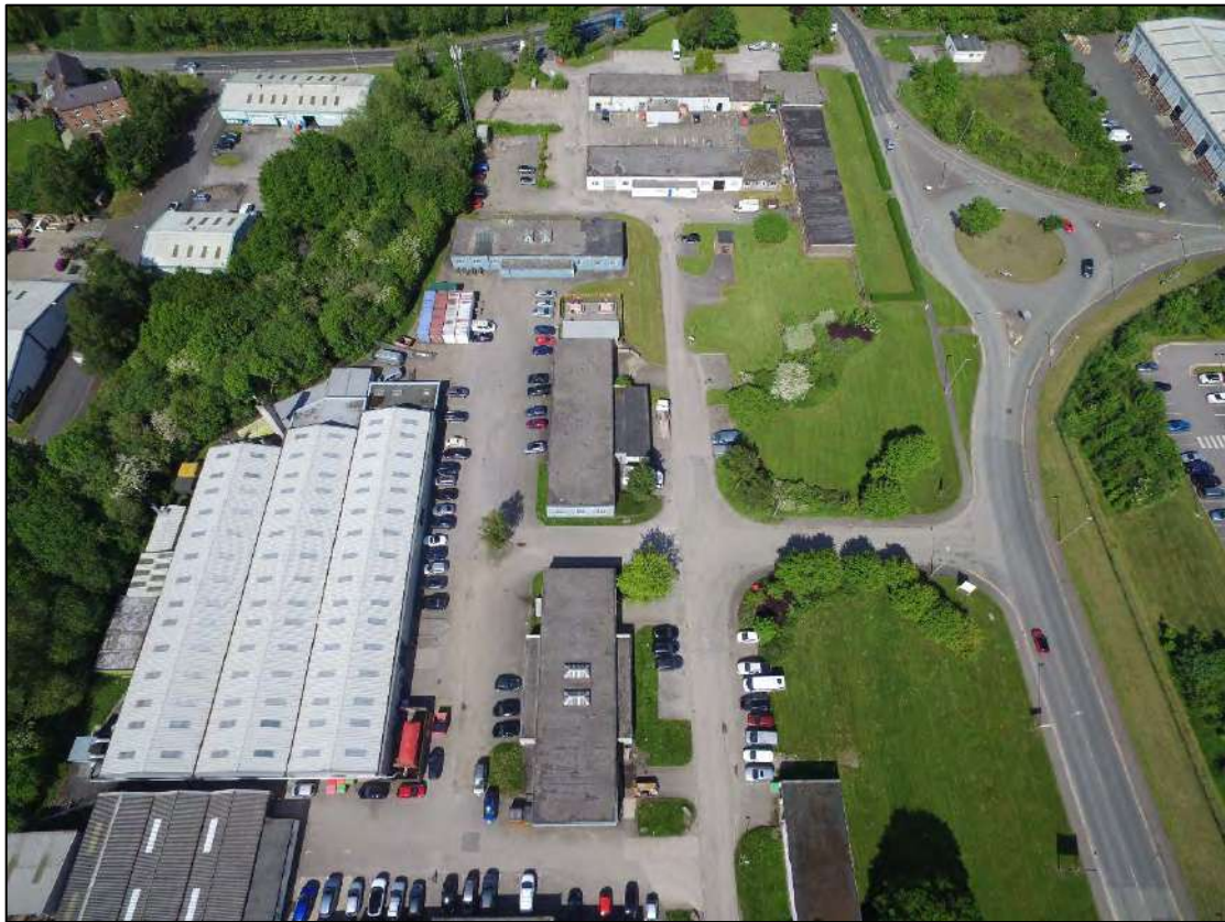
Plate 1: Recent aerial view of the of The Bridgeway centre, looking north-east across the north-east end of the Site, with Bridge Road running along the right of the picture
