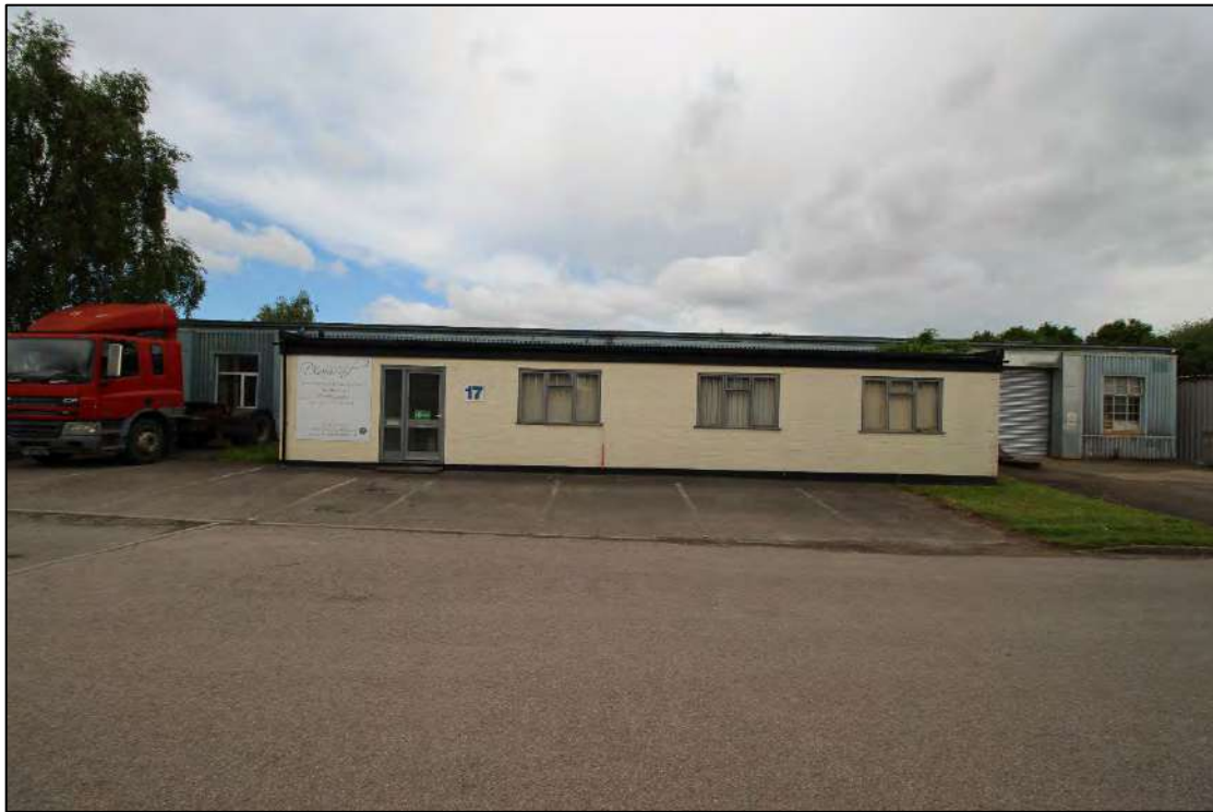
Plate 38: Later brick extension to south-east lean-to
