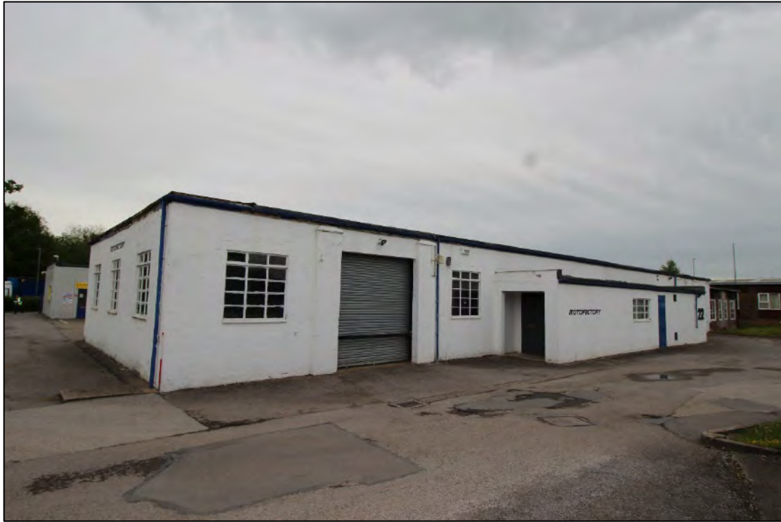
Plate 17: Principal south-west elevation of Building 2, looking east
