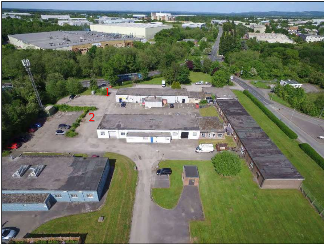
Plate 10: Recent UAV shot of Buildings 1 and 2 (indicated) with modern extensions at north-east end of the Site
