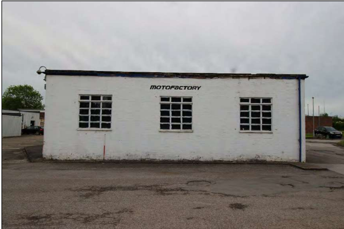
Plate 22: North-west elevation of Building 2, looking south-east
