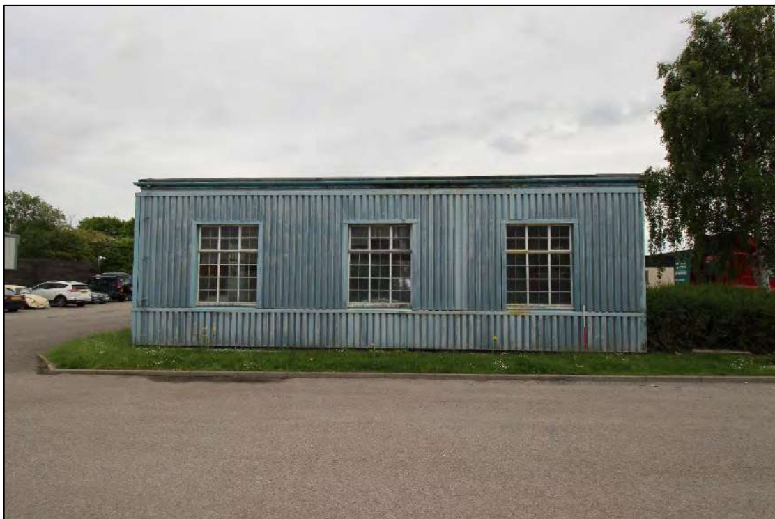
Plate 40: South-west elevation of Building 4, looking north-east
