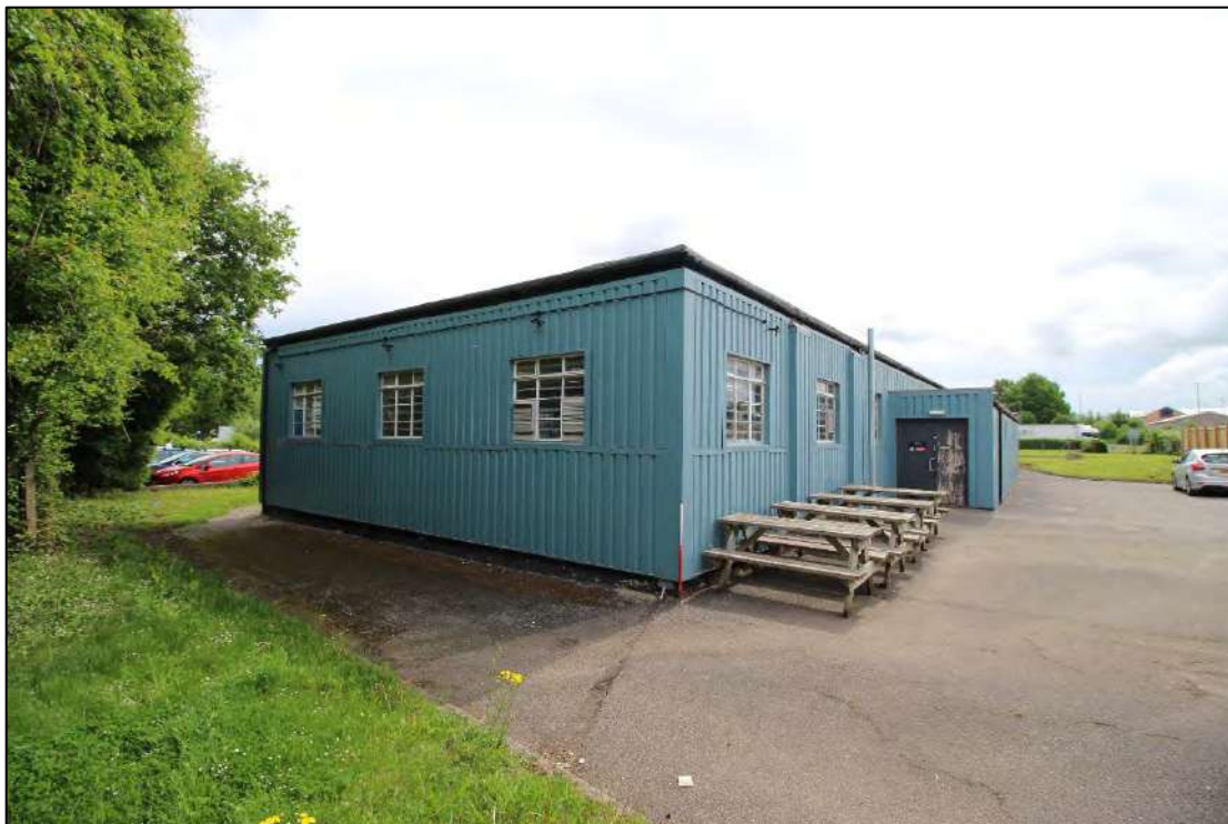
Plate 33: North-west end elevation of Building 3, looking east
