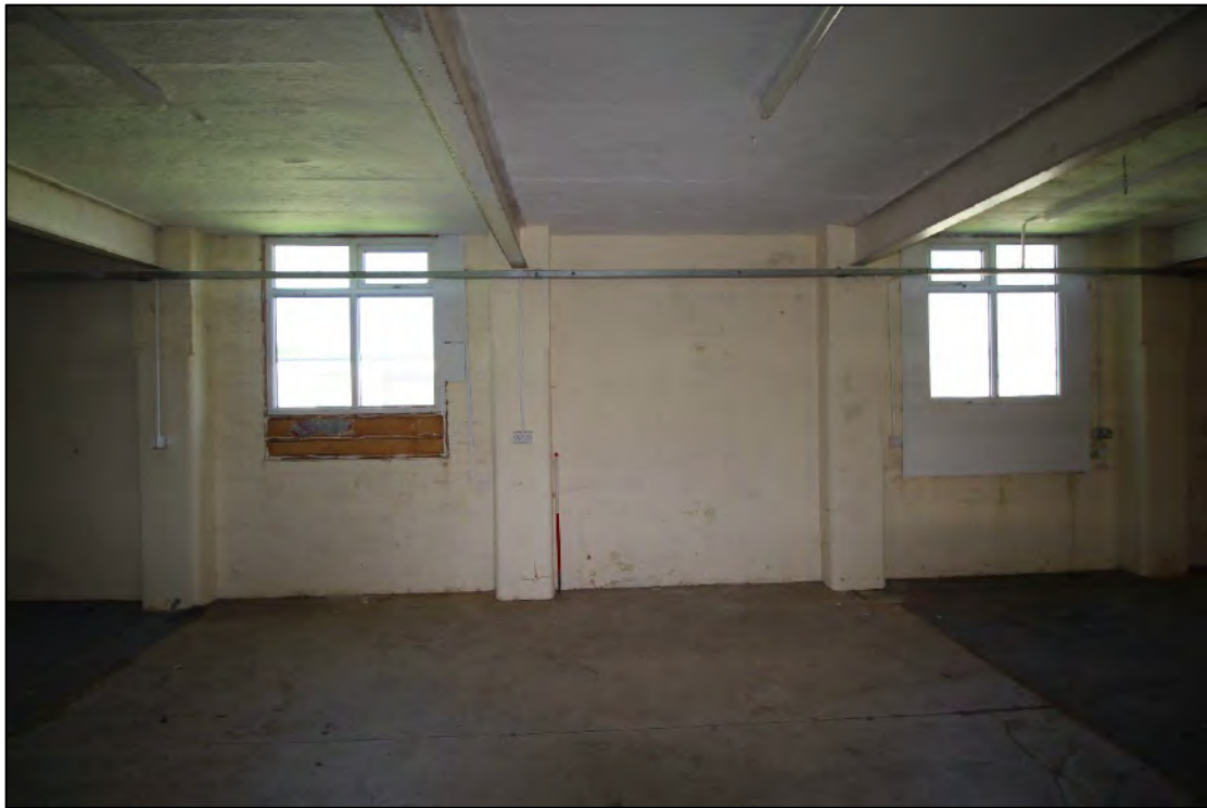
Plate 56: Remodelled windows with the front, north-west wall, looking north-west
