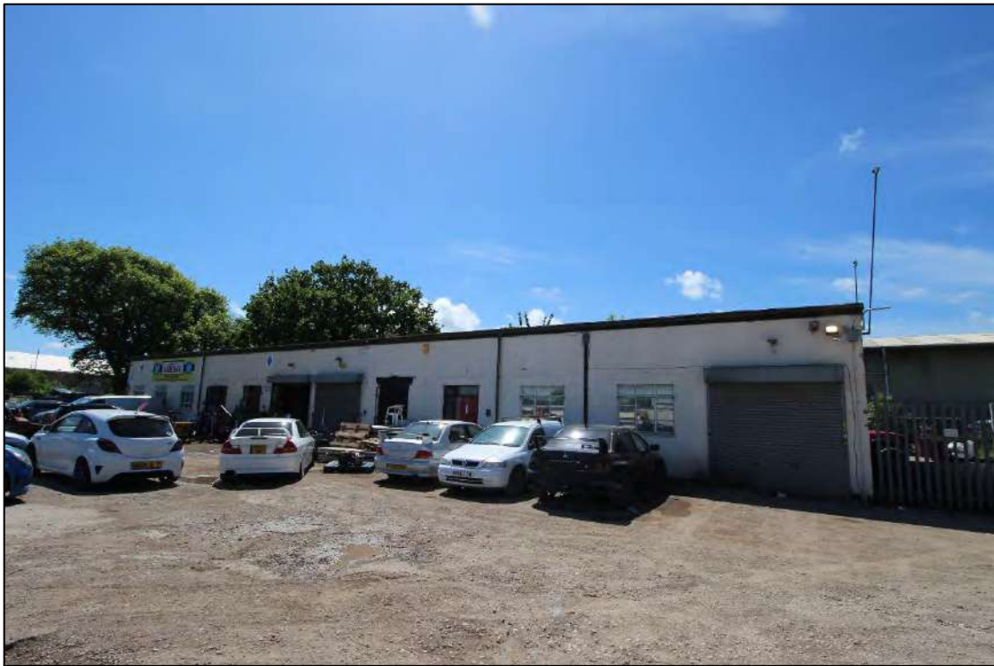
Plate 79: North-west end of north-east elevation of Building 9, looking south
