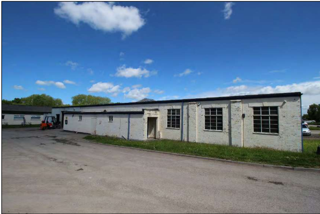
Plate 60: South-east windows bays of south-west elevation of Building 7, looking north
