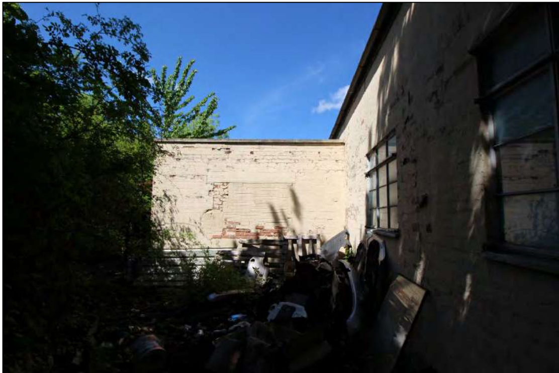
Plate 76: Blocked opening in south-east end of rear lean-to, looking north-west along rear south-west elevation
