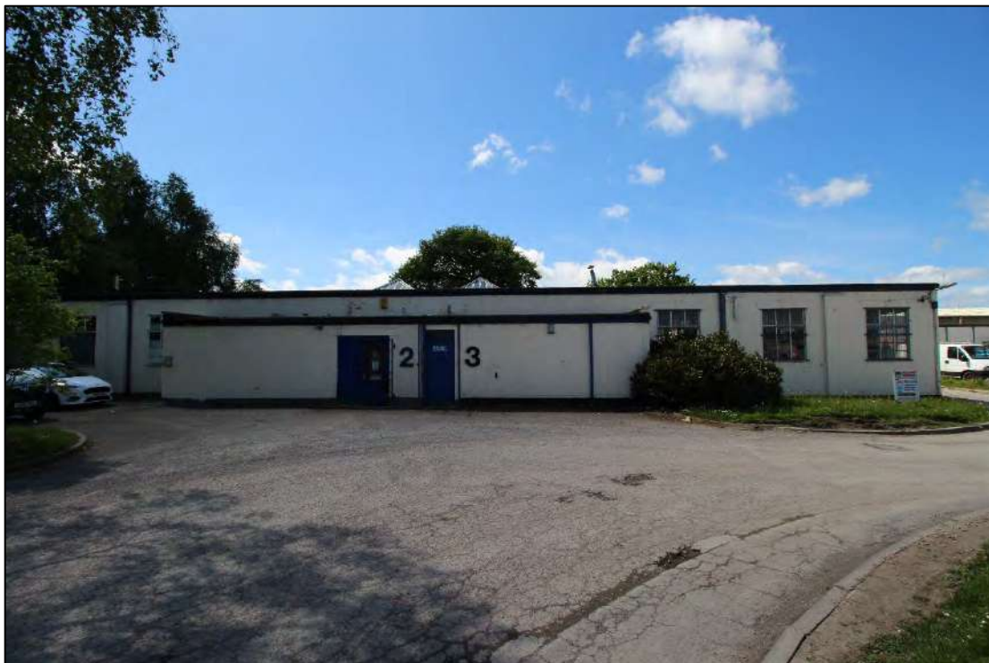
Plate 65: North-east elevation of Building 8, looking south-west across bend of service road
