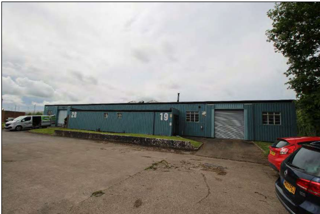
Plate 32: North-east elevation of Building 3, looking south-west
