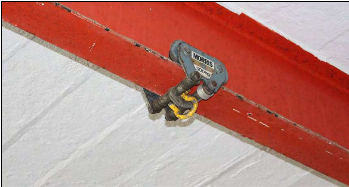
Plate 28: Detail of travelling beam trolley attached to I-beam at north-west end of Building 2
