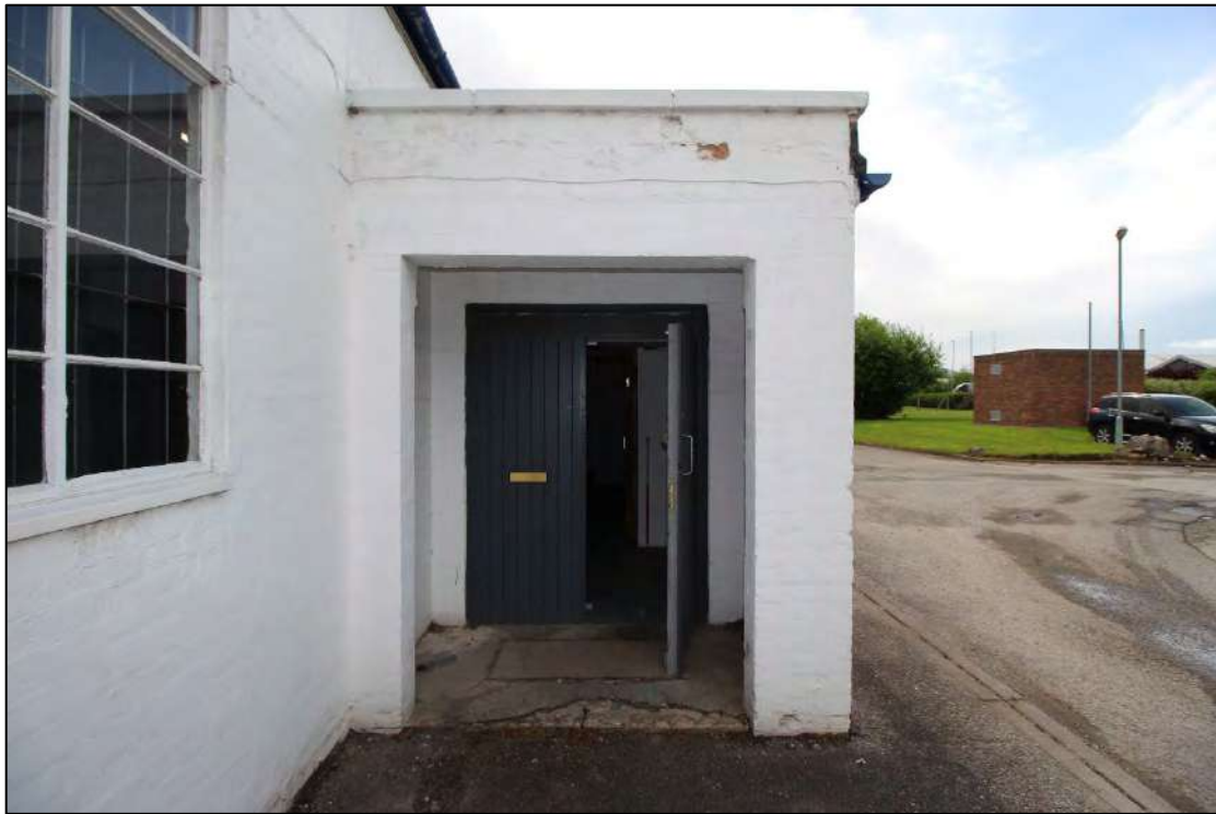
Plate 23: Entrance to north-west unit within Building 2, from south-west elevation, looking south-east
