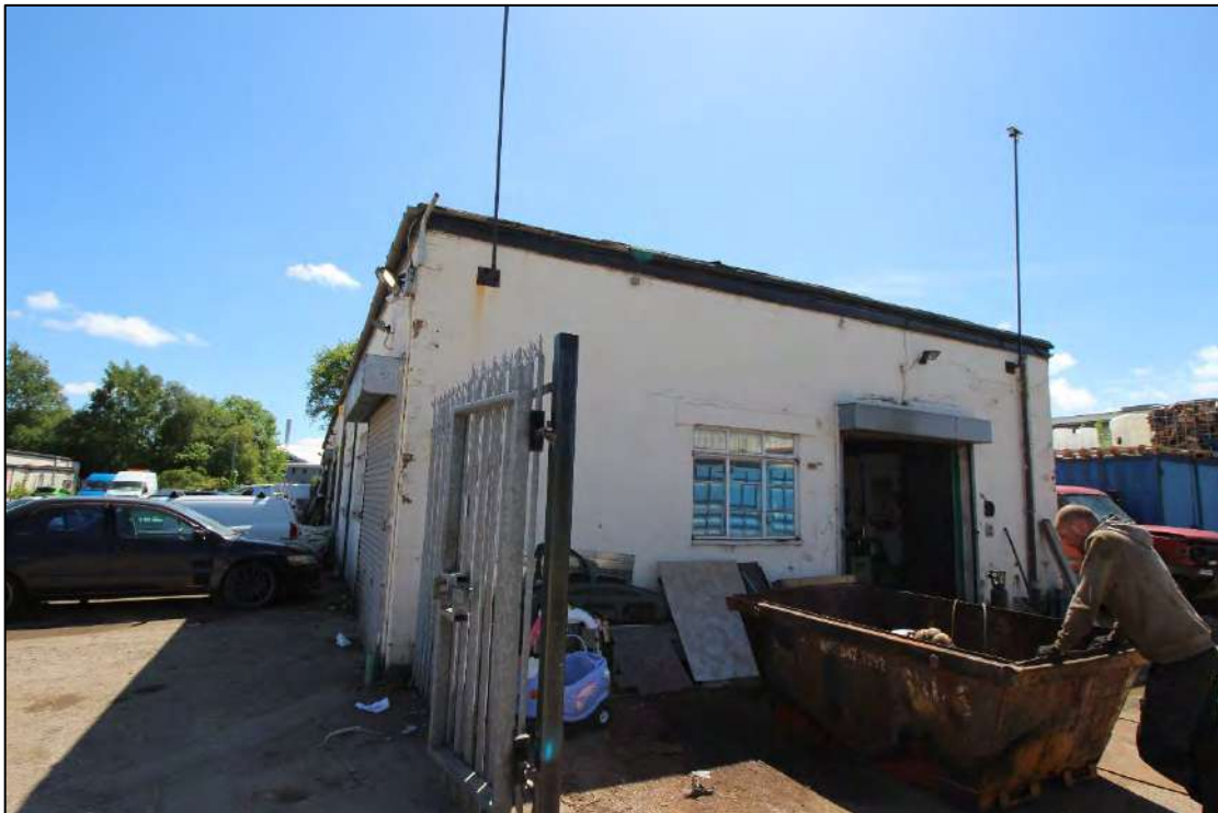
Plate 80: North-west elevation of Building 9, looking south-east
