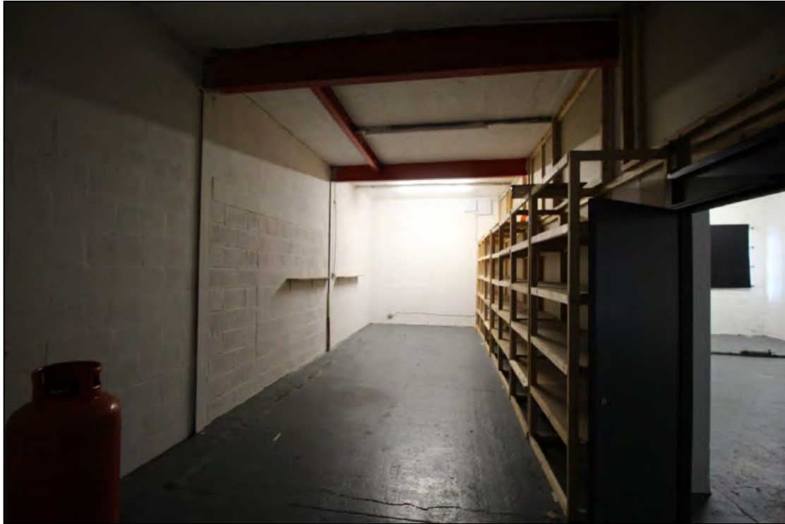
Plate 25: Inserted cinder block dividing wall across the centre of Building 2, looking south-west
