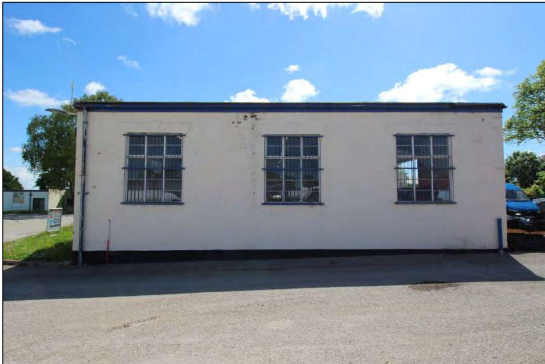
Plate 68: North-west elevation of Building 8, with examples of embellished lintels, looking south-east
