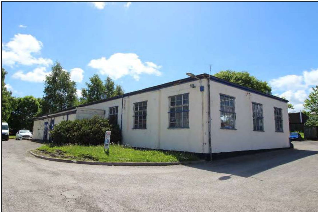
Plate 67: North-west end of north-east elevation of Building 8, looking south
