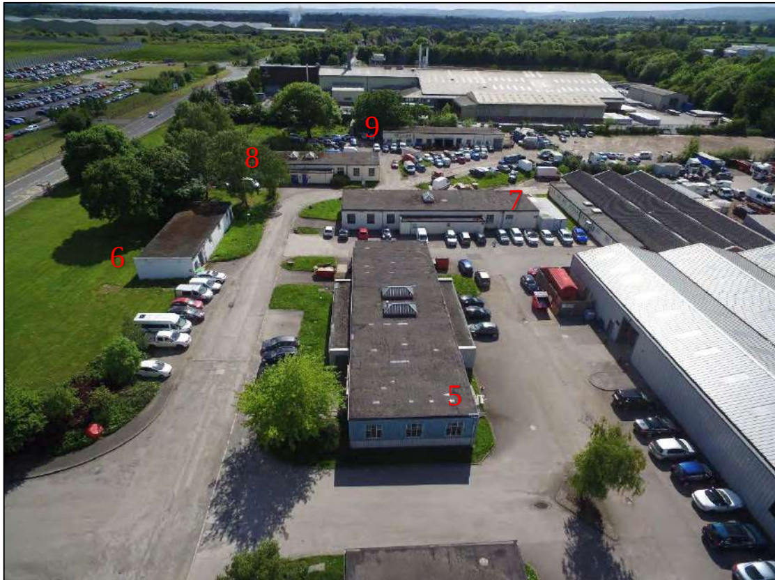
Plate 58: Recent UAV view of south-west site of the Site with buildings indicated, looking south-west
