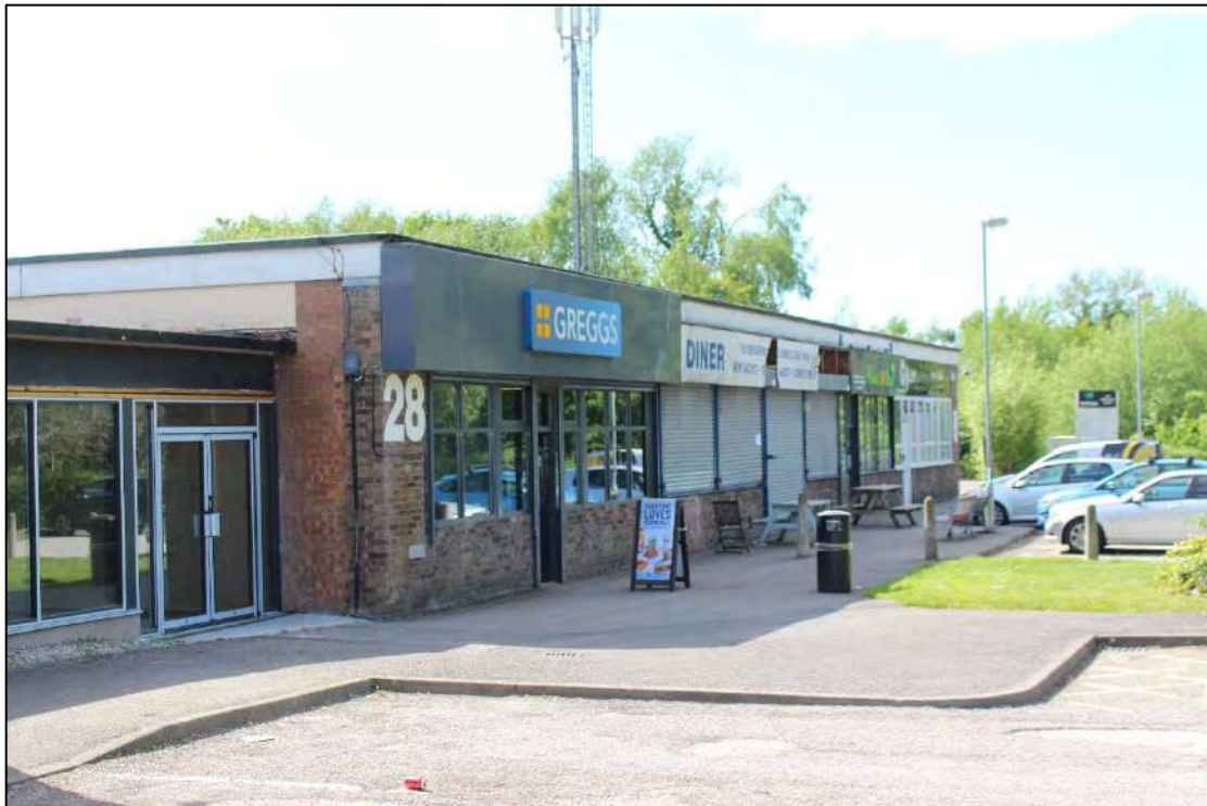
Plate 11: North-east elevation of Building 1, looking west.
