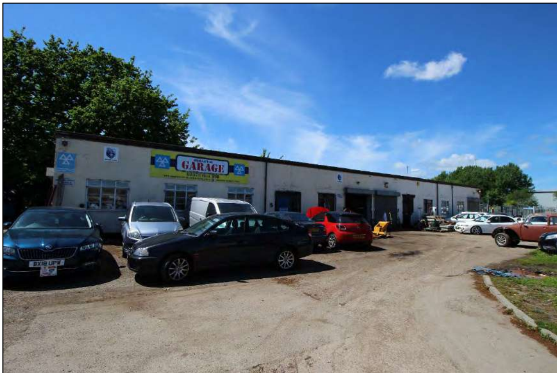
Plate 78: Front north-east elevation of Building 9, looking west
