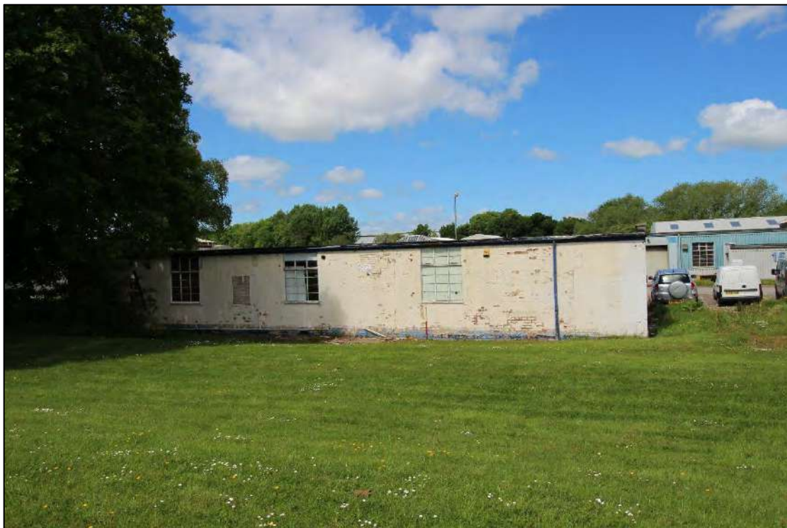
Plate 53: Rear, south-east elevation of Building 6, looking north-west from verge of Bridge Road
