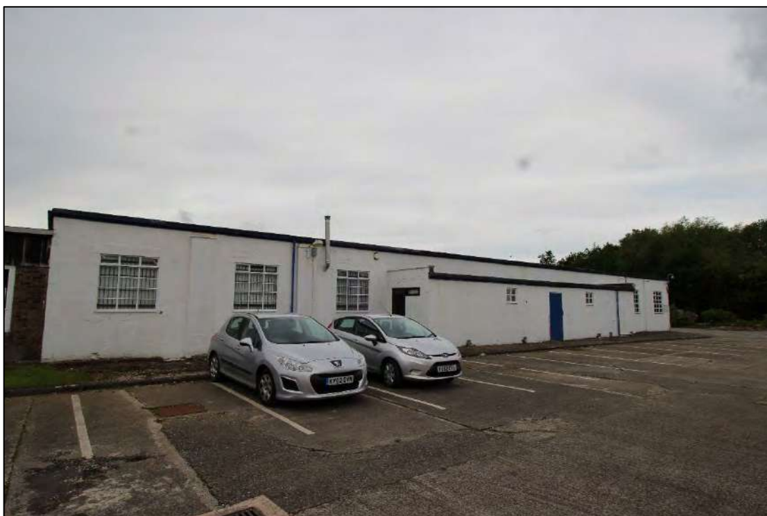
Plate 19: Window bays within the north-east elevation of Building 2, looking west
