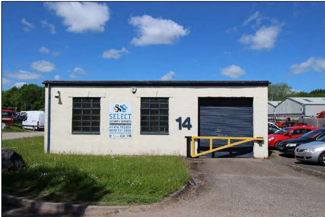
Plate 61: South-east elevation of Building 7, looking north-west
