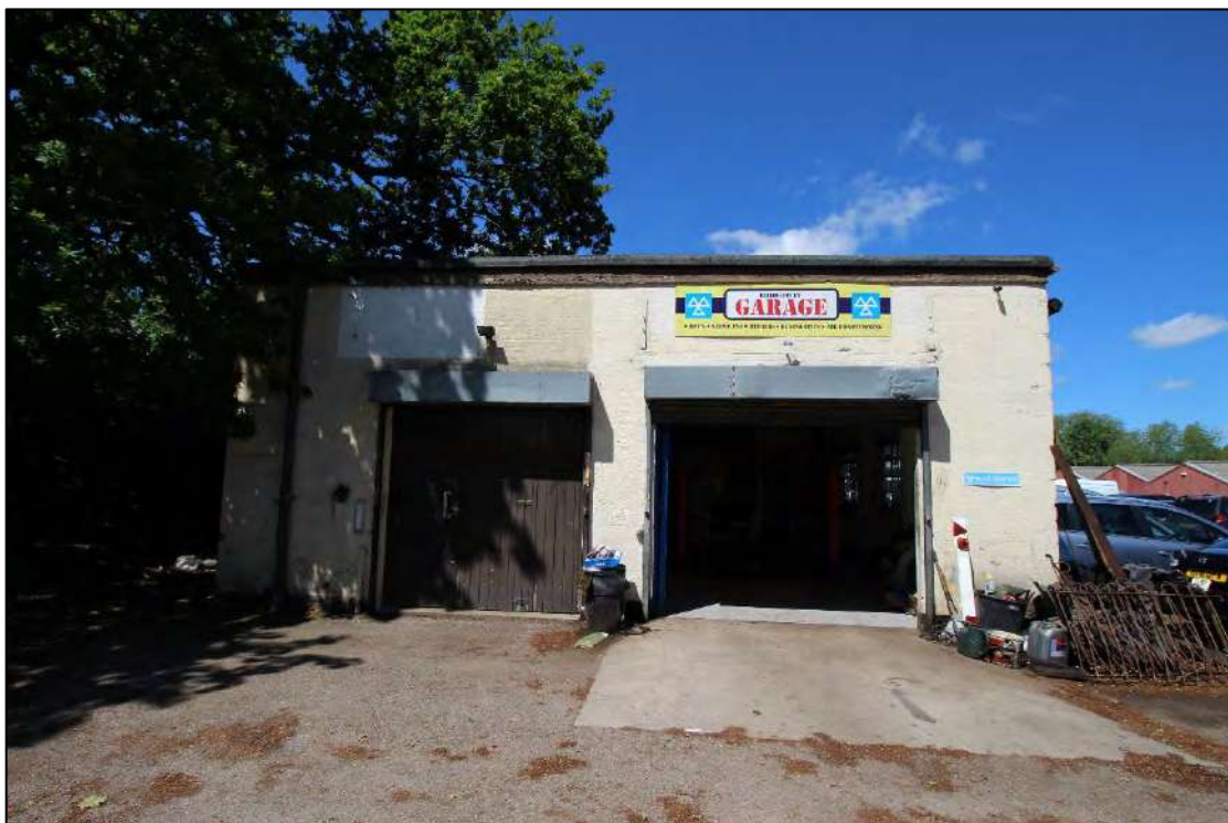
Plate 77: Vehicle entrances in south-east elevation of Building 9
