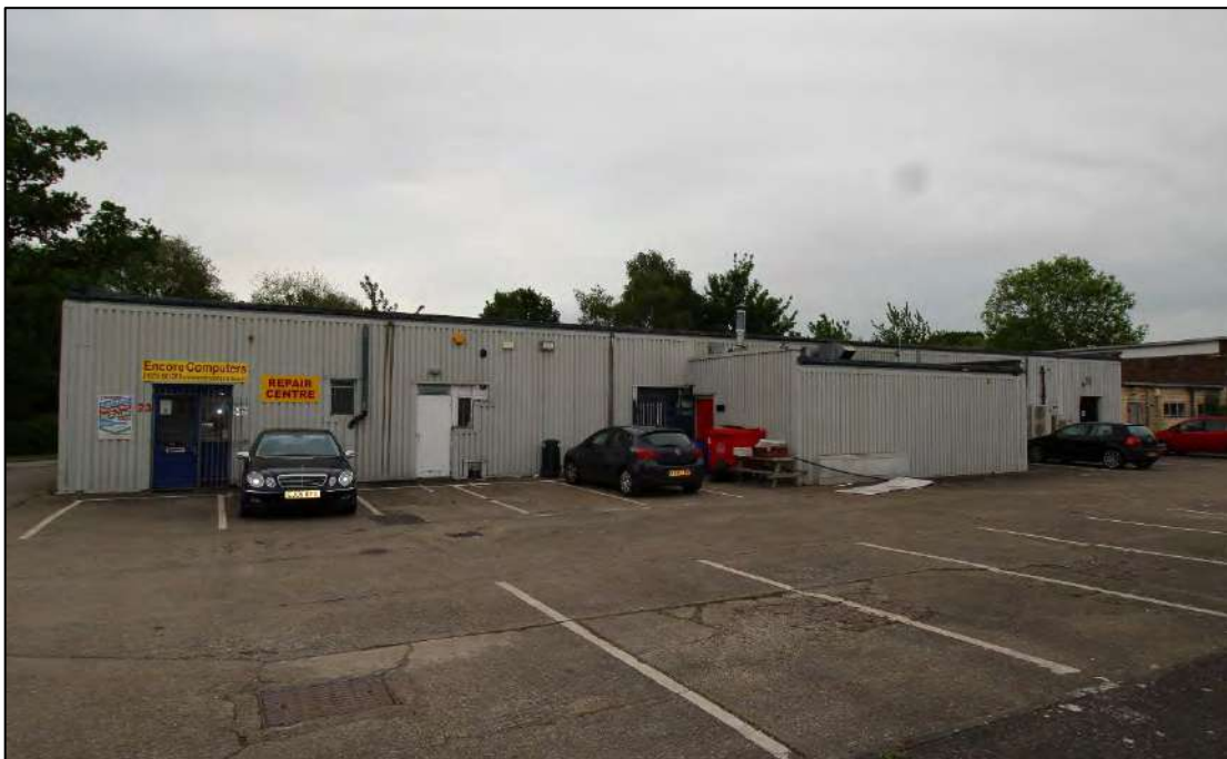
Plate 13: Rear, south-west elevation of Building 1, looking north-east
