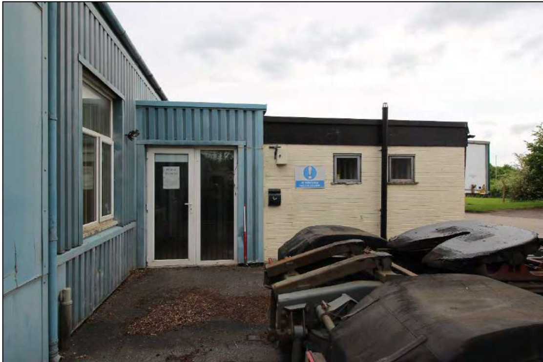
Plate 37: Modern extension to lean-to on front, south-east elevation, looking north-east
