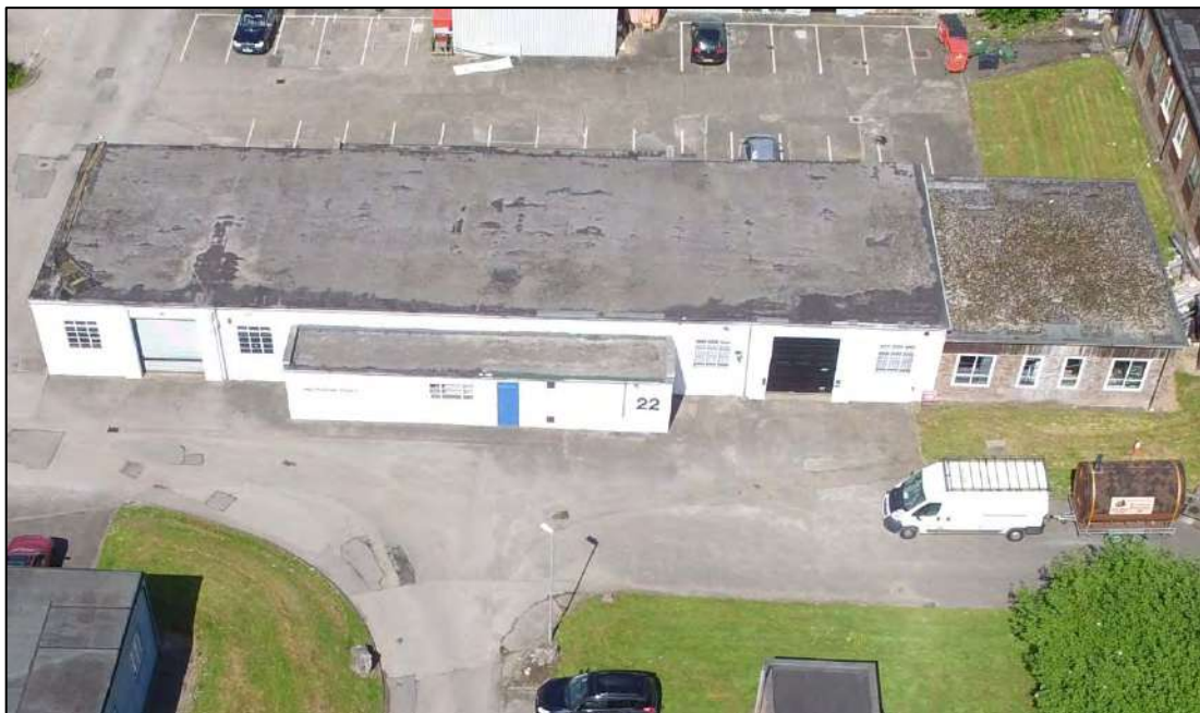
Plate 16: Recent UAV photograph of Building 2 with modern extension, looking north-east
