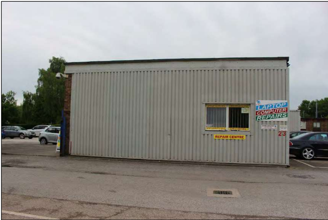
Plate 12: North-west end elevation of Building 1, looking south-east
