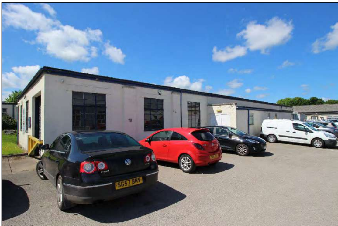
Plate 62: Rear north-east elevation of Building 7, looking west
