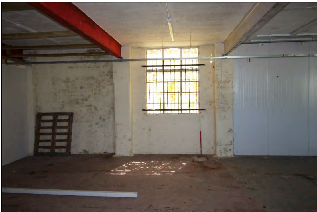
Plate 57: Tall, steel framed window within rear, south-east wall
