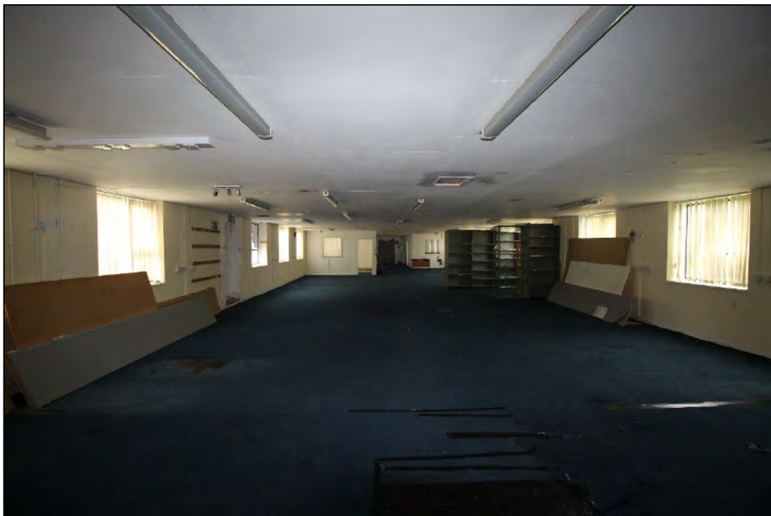
Plate 15: Interior of modern office range adjacent to Building 1
