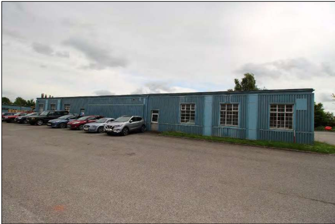
Plate 41: Rear, south-west elevation of Building 4, looking east
