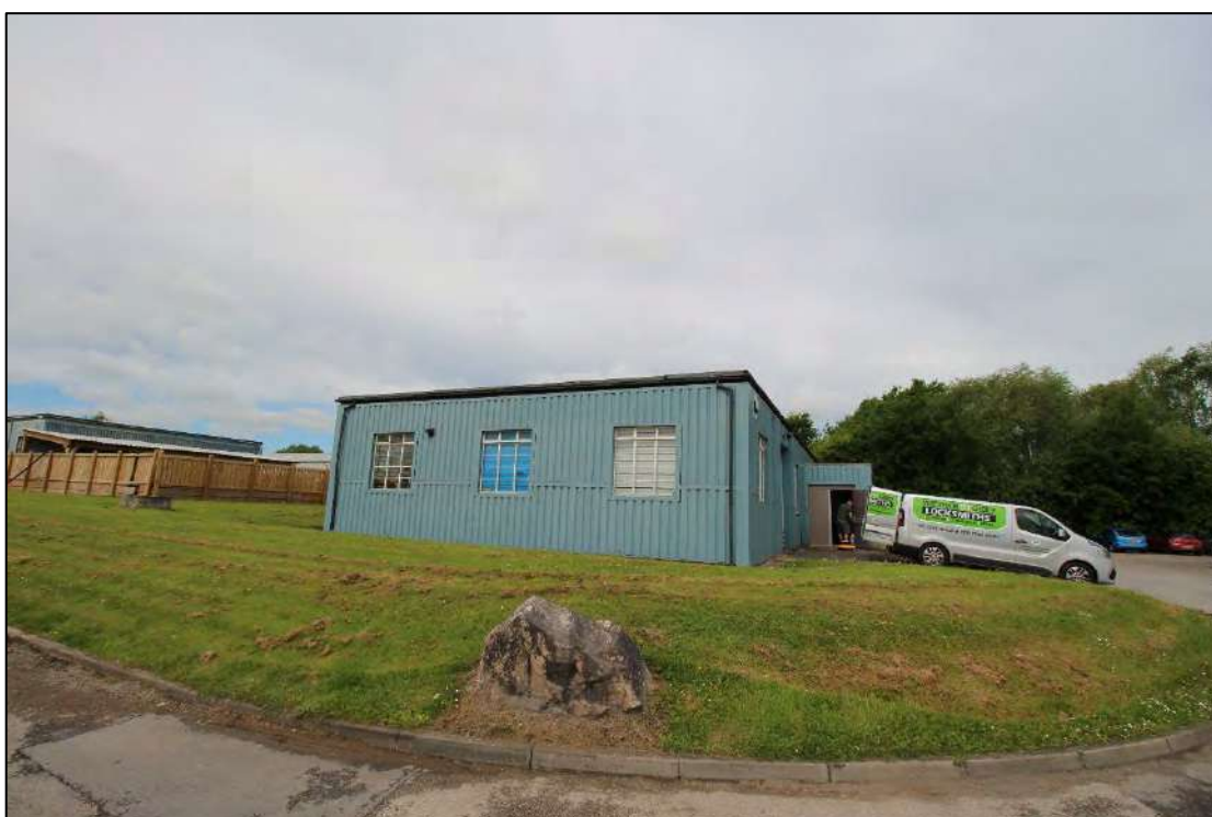
Plate 34: South-east end elevation of Building 3, looking north-west
