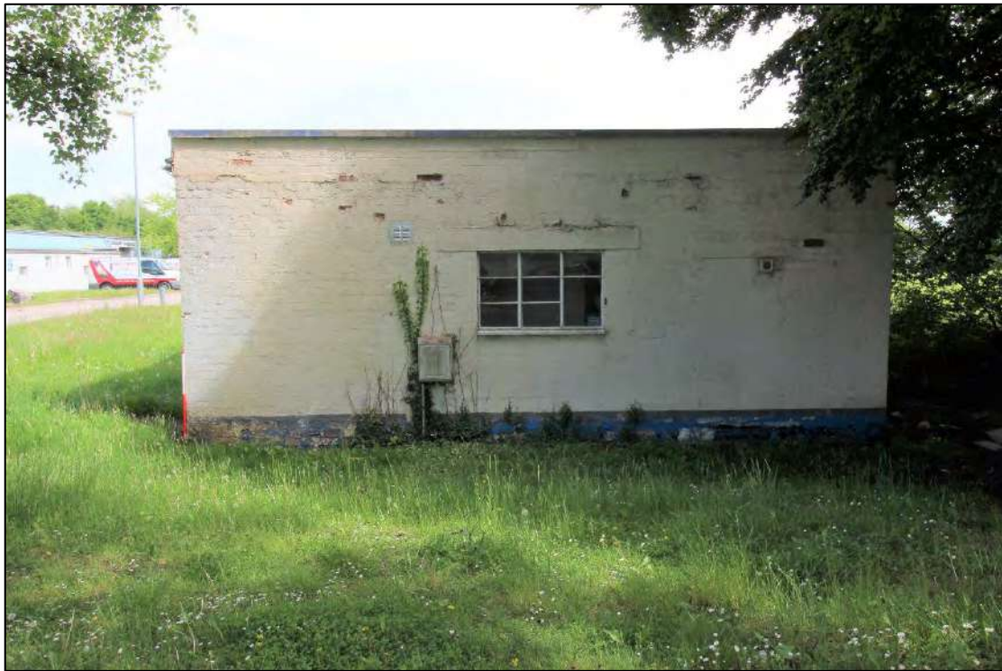
Plate 52: Remodelled openings with south-west elevation of Building 6
