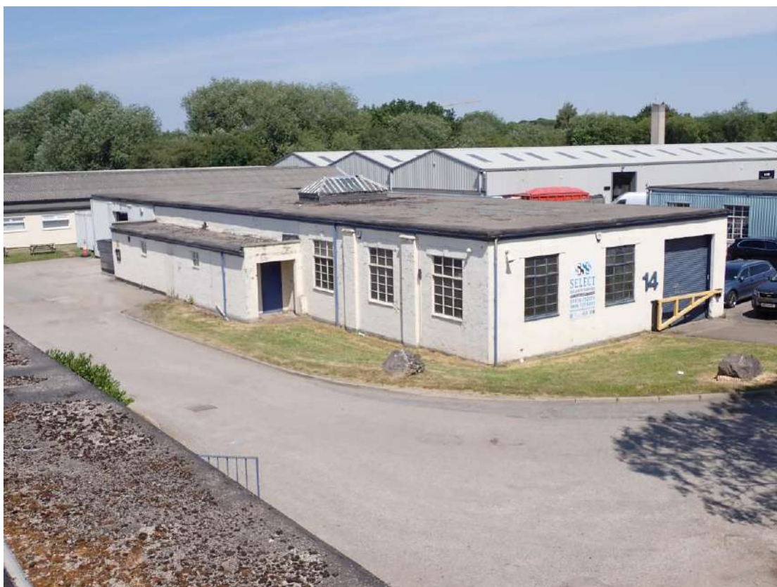
Photograph 10 – Southern aspect of Building 3.
