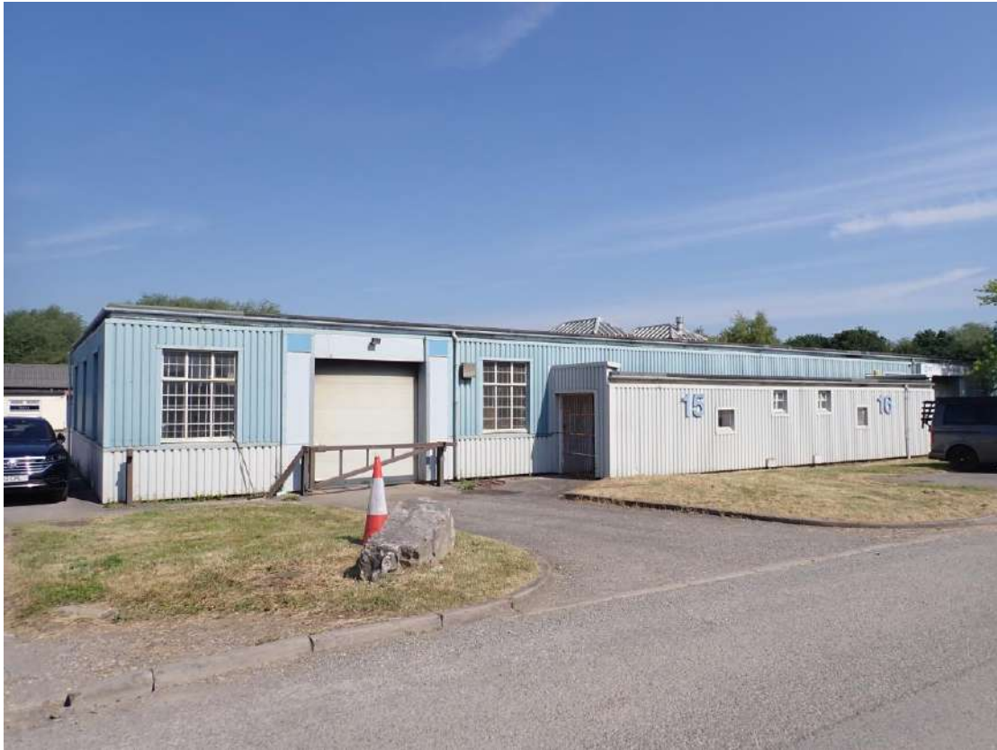
Photograph 1 – Southeastern aspect of Building 1.
