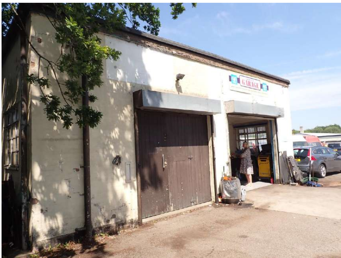
Photograph 21 – Southeastern aspect of Building 5.
