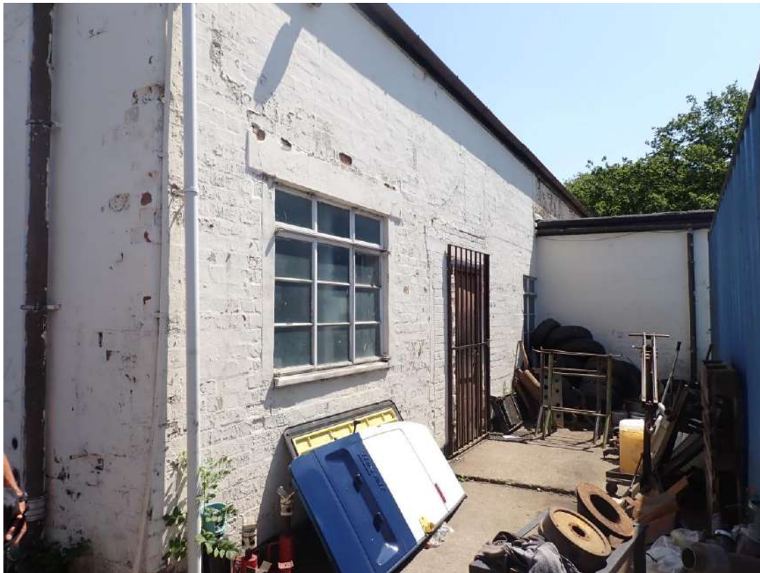
Photograph 25 – Southwestern aspect of Building 5 (further West than Photograph 16).
