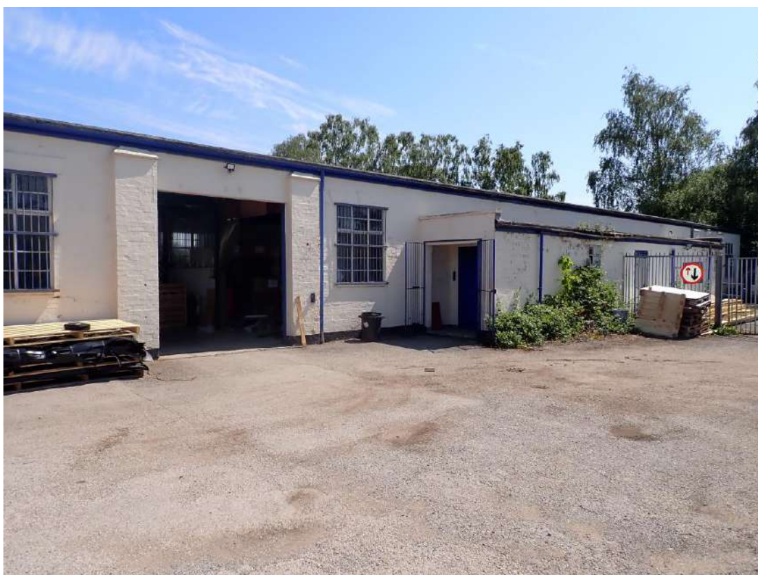
Photograph 14 – Southwestern aspect of Building 4.
