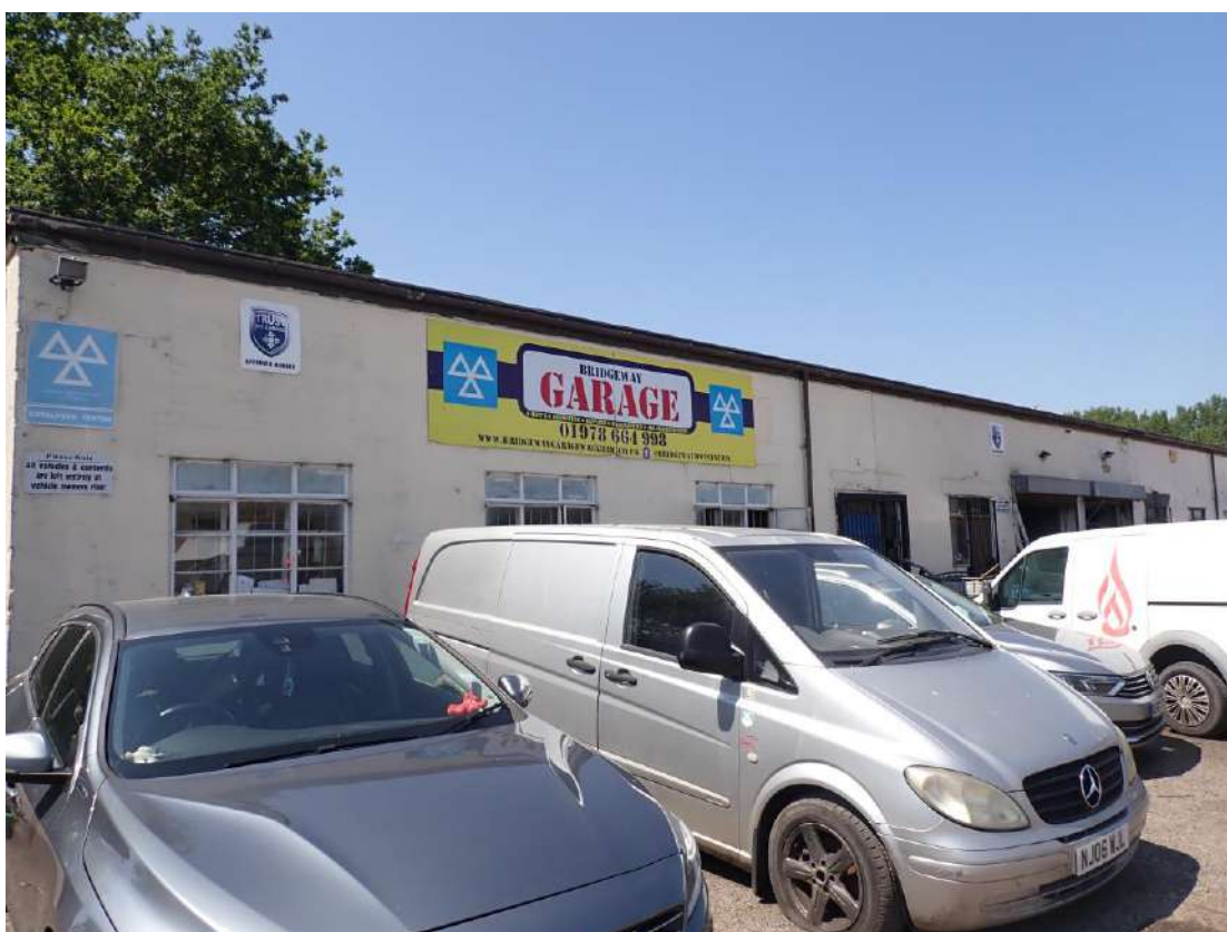
Photograph 22 – Northeastern aspect of Building 5.
