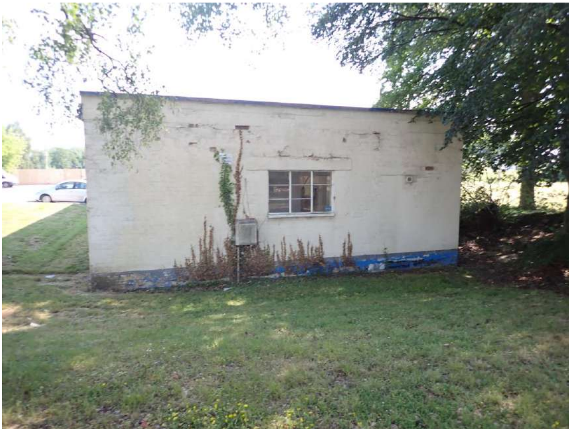
Photograph 8 – Southwestern aspect of Building 2.
