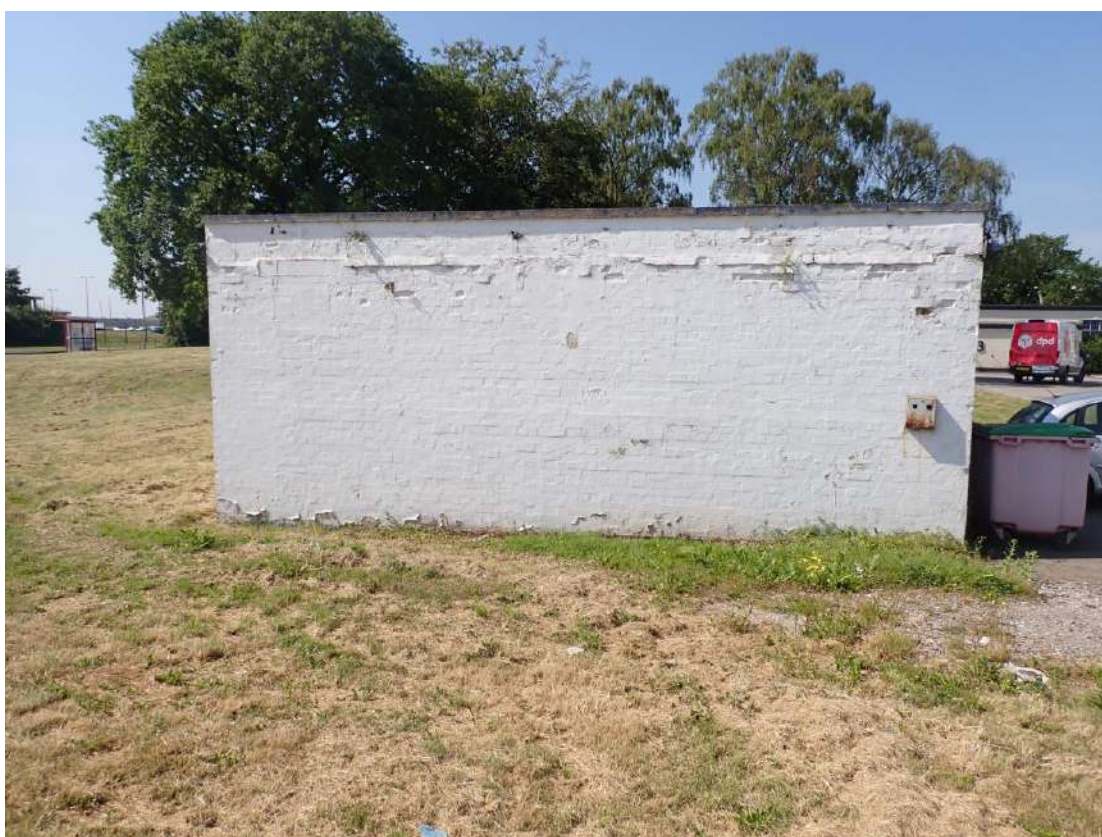
Photograph 6 – Northeastern aspect of Building 2.
