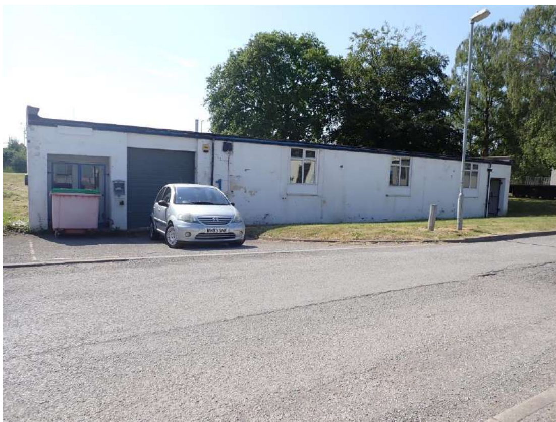
Photograph 5 – Northwestern aspect of Building 2.
