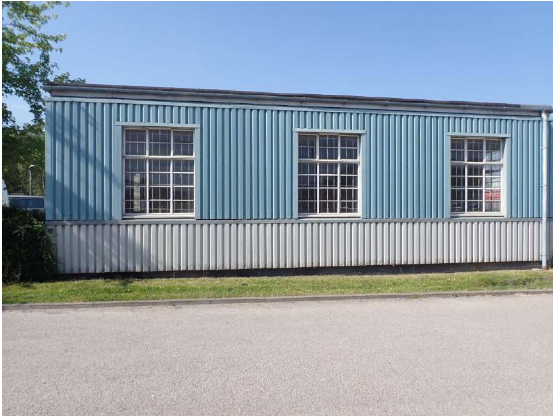
Photograph 3 – Northeastern aspect of Building 1.
