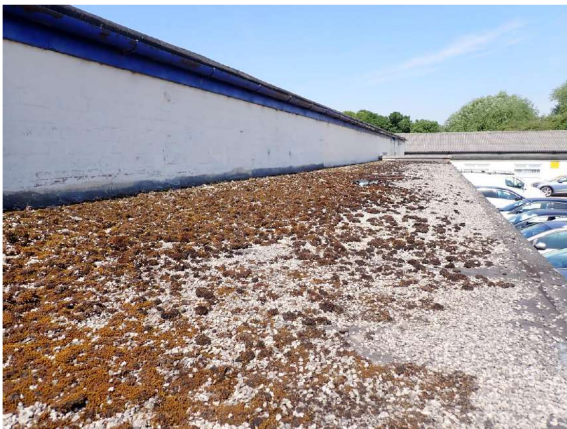
Photograph 13 – Northeastern aspect of Building 3.
