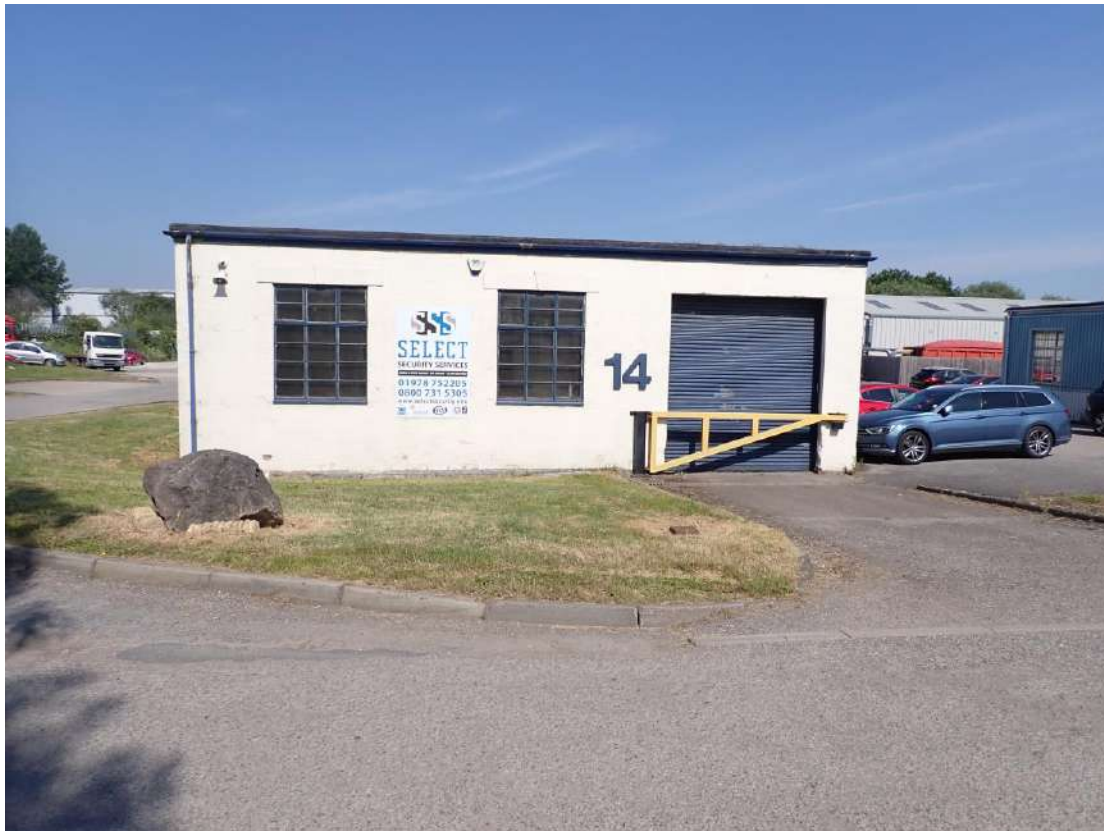
Photograph 9 – Southeastern aspect of Building 3.
