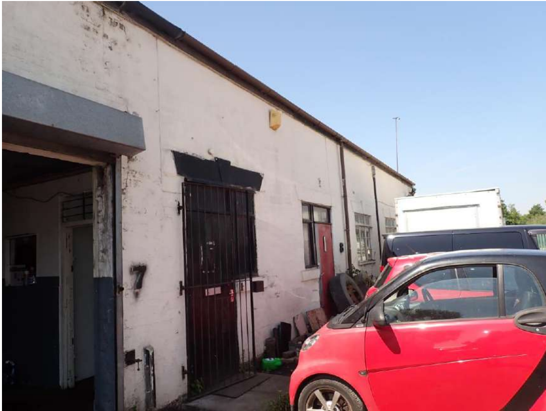
Photograph 23 – Northeastern aspect of Building 5 (further north than Photograph 18).
