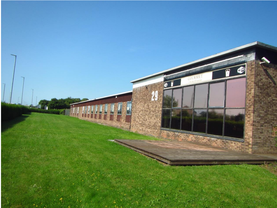
Photograph 1 – Eastern aspect of Building 1.
