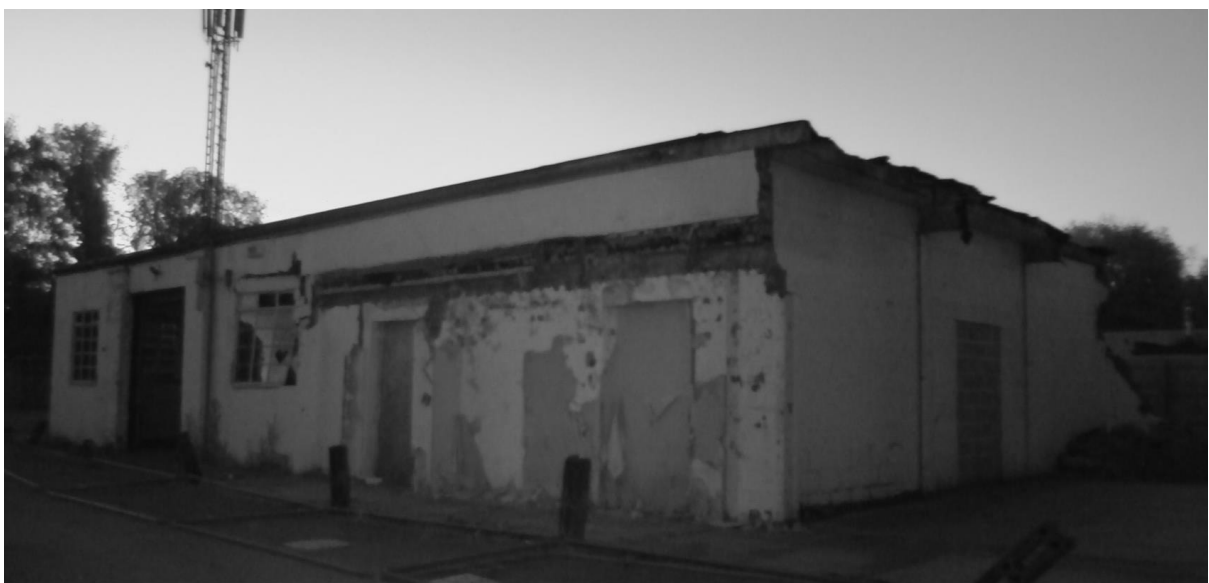
Camera Viewpoint 6 – Southwestern aspect of Building 2 on 17/06/2024.
