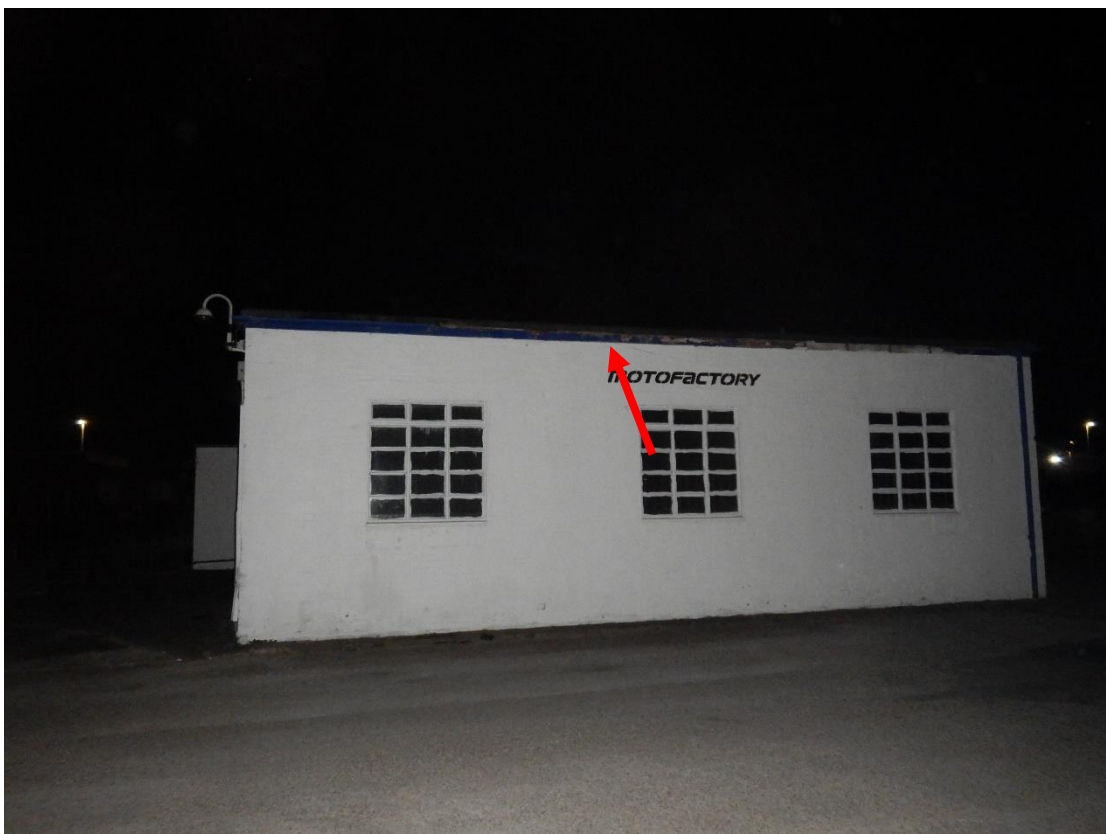
Photograph 6 – Western aspect of Building 2, showing the location of Roost 2.
