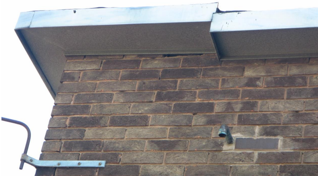
Photograph 4 - Gap in brickwork on southern aspect of Building 1.
