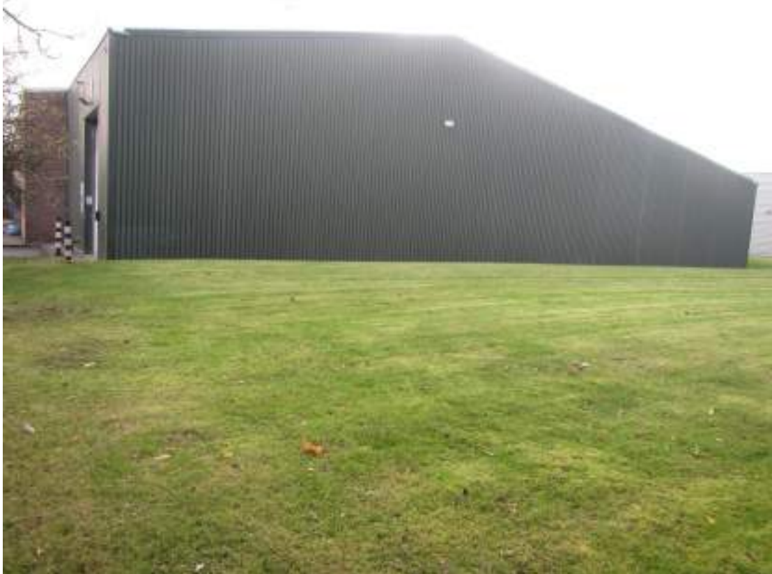
Photograph 8 – View of building immediately adjacent to the proposed development site boundary.
