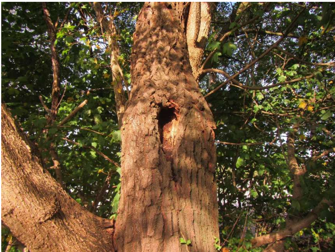
Photograph 28 – Newly identified bat potential roosting feature within field maple tree in the southern section of the site.
