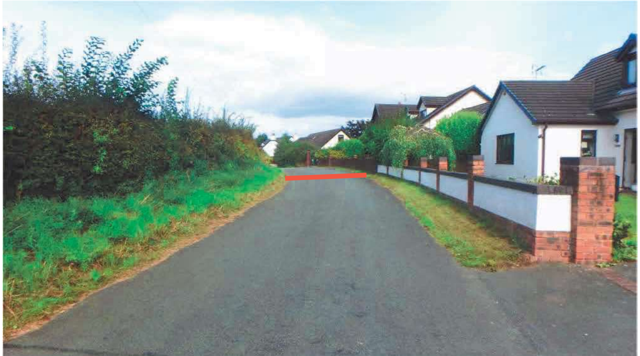
PHOTOGRAPH 7 The red line is 96.0m from the access where the road width is 4.5m
