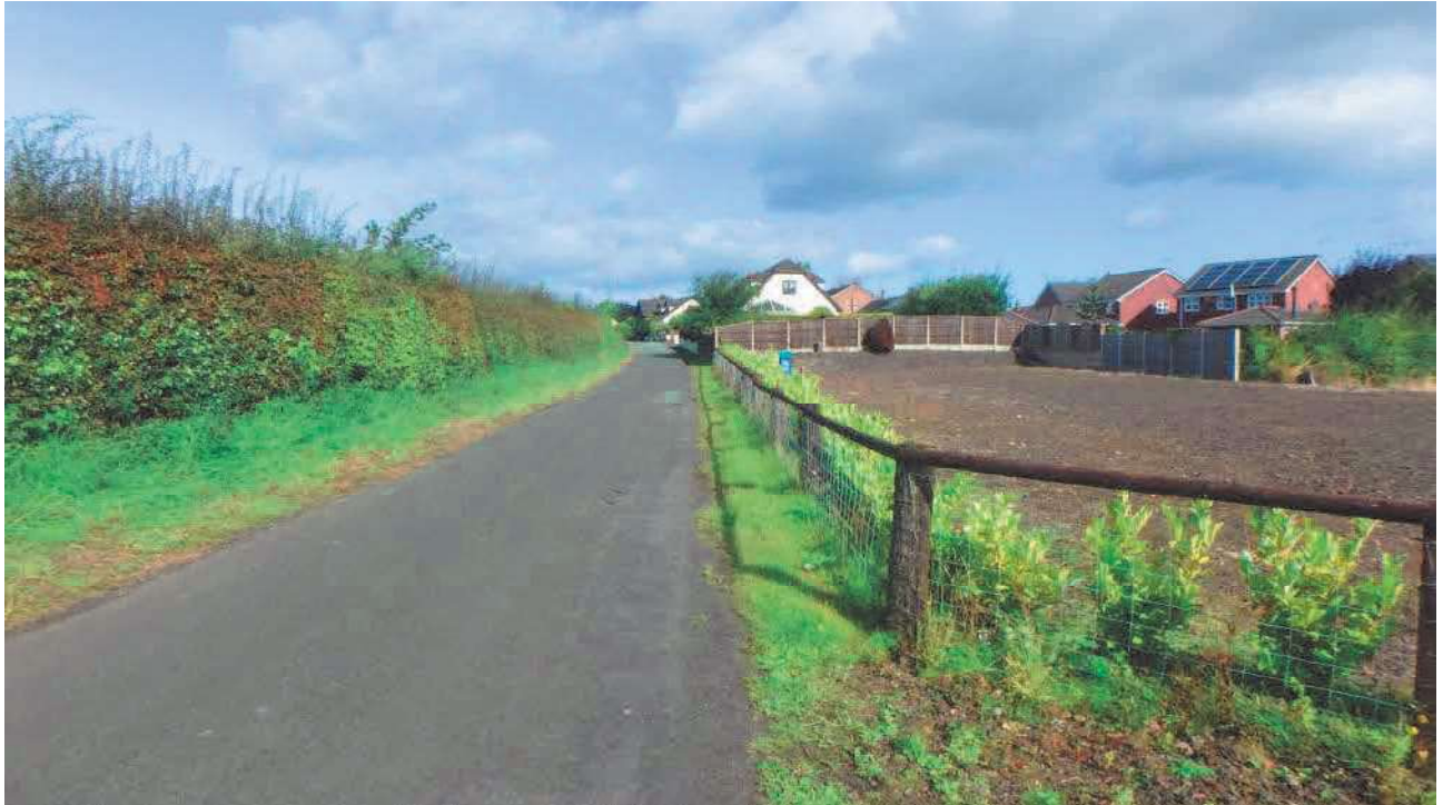
PHOTOGRAPH 3 Road channel at the access looking in a north-westerly direction
