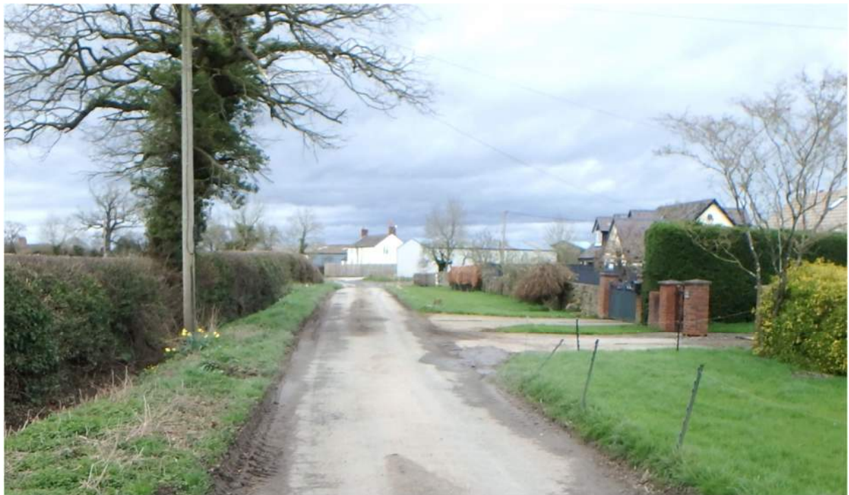
PHOTOGRAPH 8 PPP 18 Looking north
