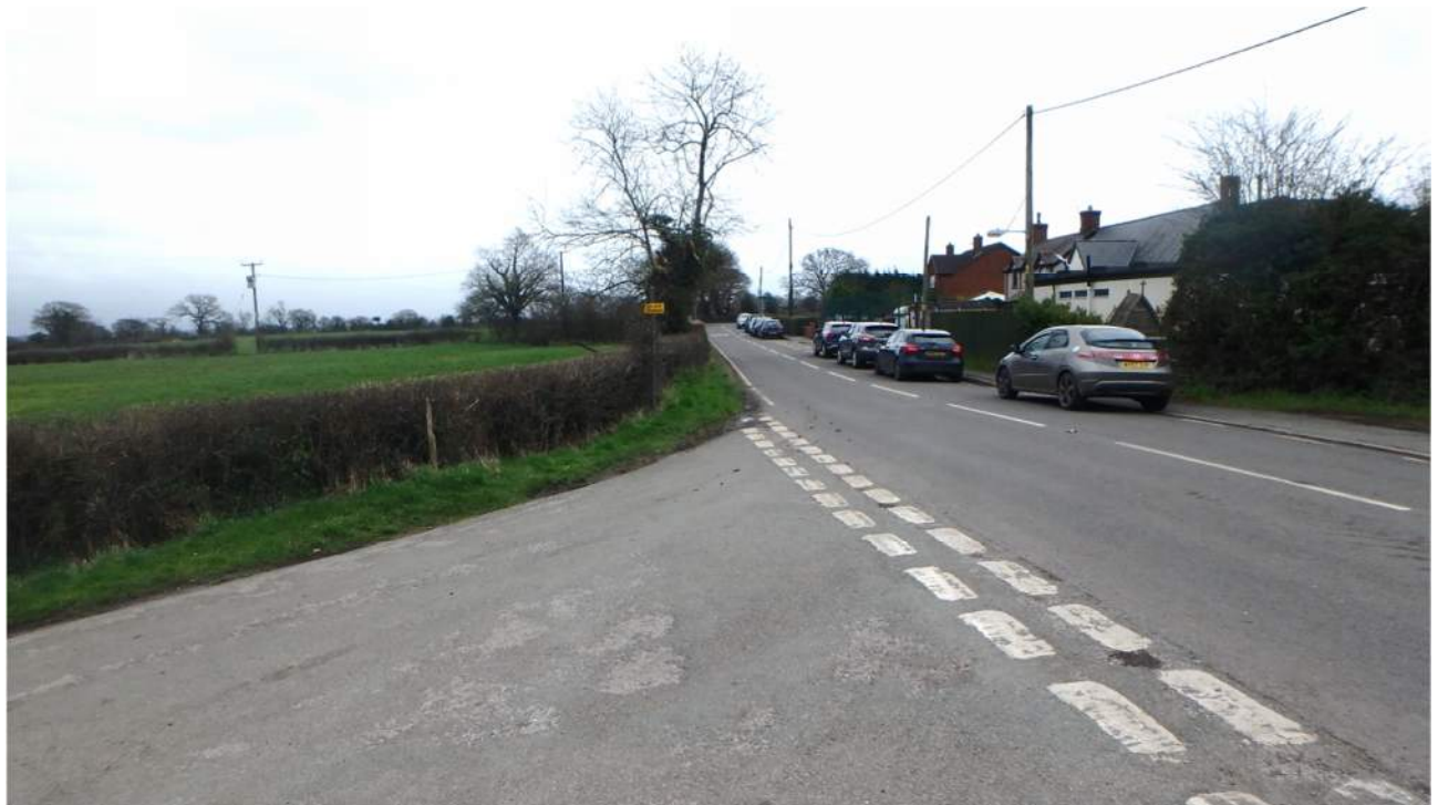
PHOTOGRAPH 18 B5130 Northern Junction at 2.4m to the left (south)
