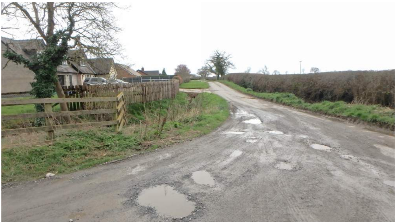
PHOTOGRAPH 22 Site Access at 2.4m to the left (south)
