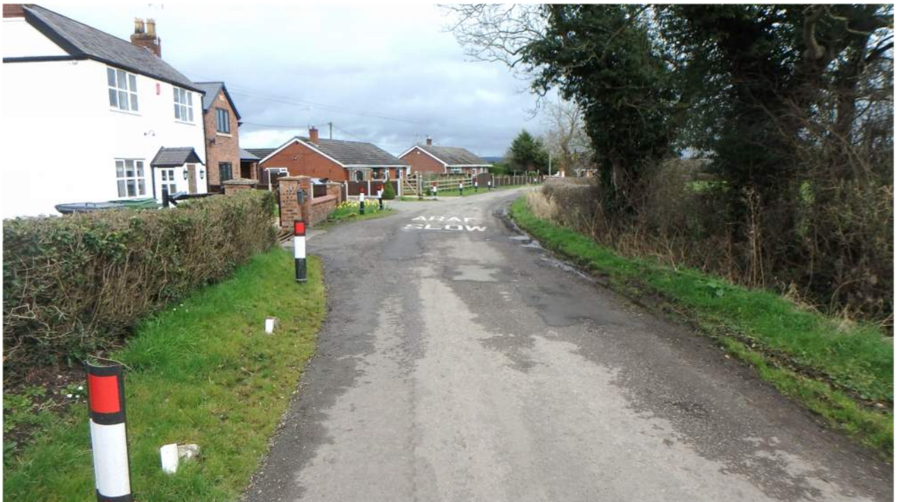
PHOTOGRAPH 2 PPP 5 & 6 Looking east
