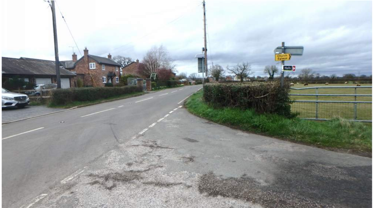
PHOTOGRAPH 17 B5130 Northern Junction at 2.4m to the right (north)
